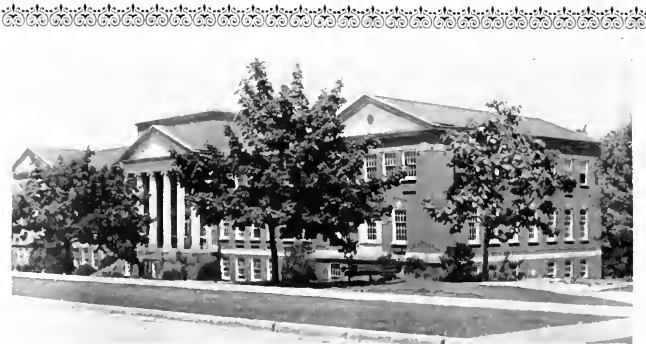
Science Building — erected in 1939
