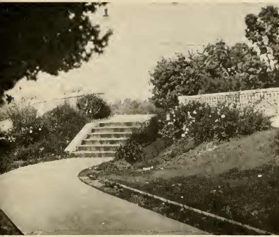
"SIX STEPS UP AND TWELVE ACROSS" (The bridge over Walker Avenue)
