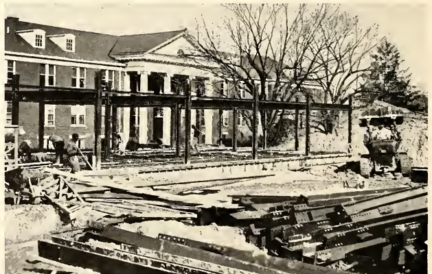
CONSTRUCTION WORK ON THE NEW LIBRARY Spencer Hall in the background
