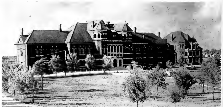
Administration Building THEN . . . and NOW
