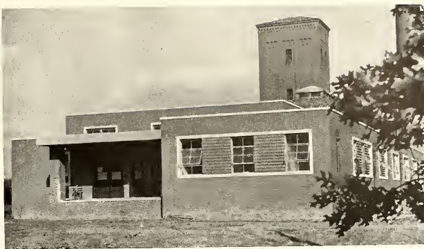
The new laundry at Woman's College which was opened this fall. It is located back of Curry Building, next to the power plant.
