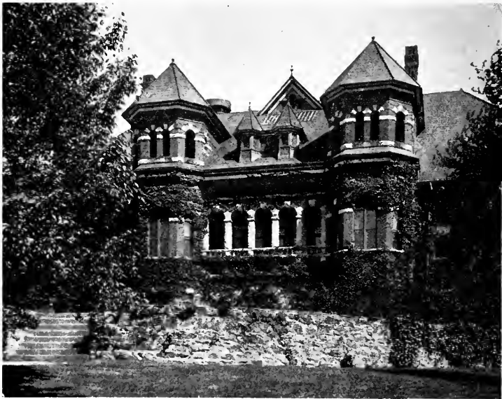
Administration Building — Now Being Remodeled
