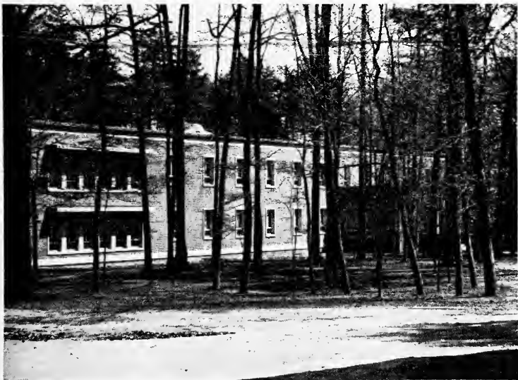
The new Anna M. Gove Infirmary which will probably be ready for use in the Fall. The building is located in the wooded section northeast of Weiland and north of Mendenhall-Ragsdale Halls.
