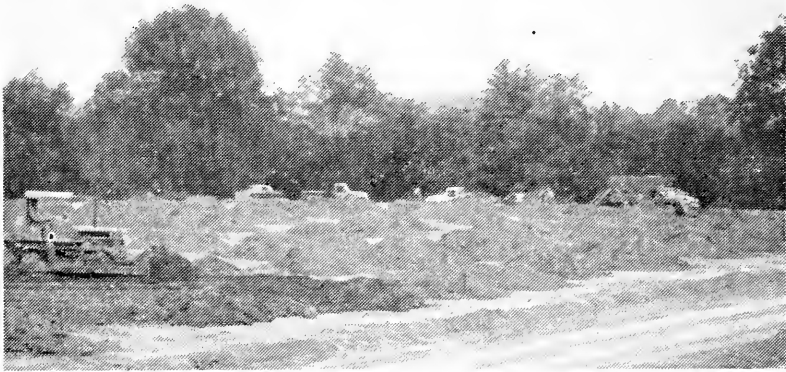
Dirt moving activity on the New Athletic Field.
