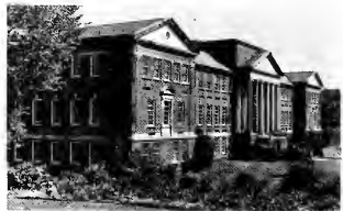
Students entering in 1940 were the first to climb the twin curving stairways leading to Petty Science Building, named after Mary Petty, head of the chemistry department for 40 years.
