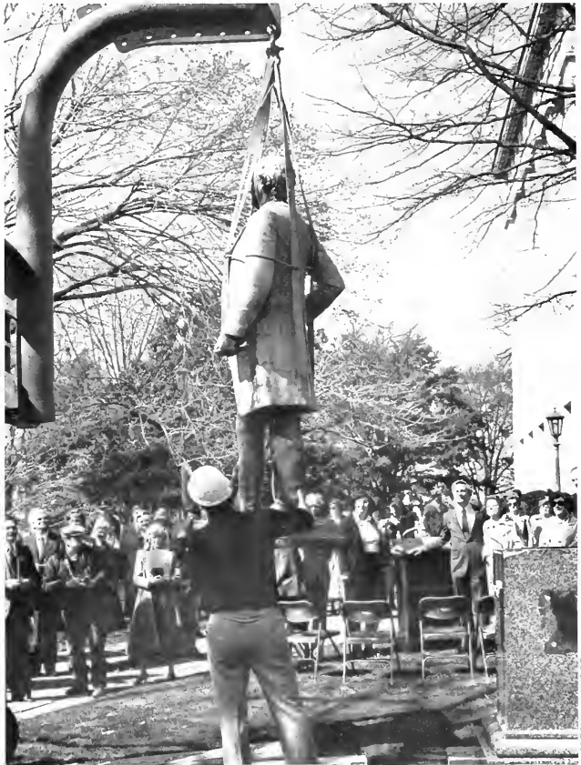
Removal of the Charles D. McIver statue for restoration, State Capitol grounds, March 9, 1982. Eleftherios Karkadoulis (back to camera) restored the statue in his foundry in Cincinnati, Ohio.
