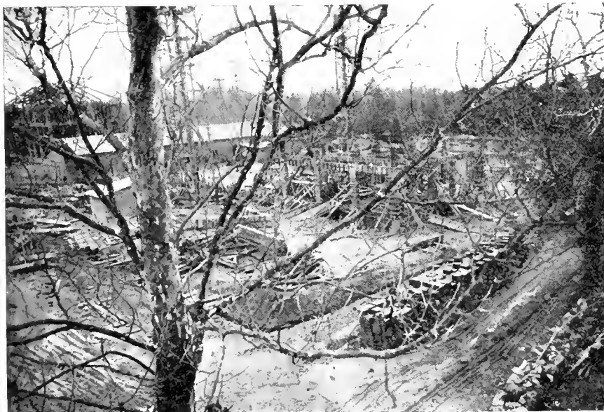
A VIEW OF THE CONSTRUCTION WORK FROM EMERSON STADIUM
