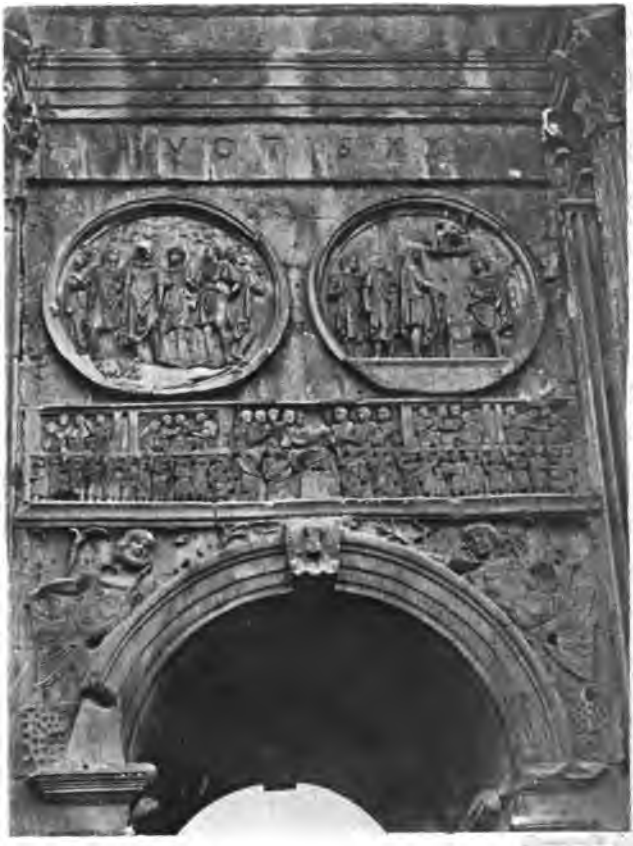
Detail of the Arch of Constantine
