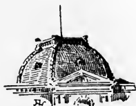
Central Pavilion of the Tuileries.
