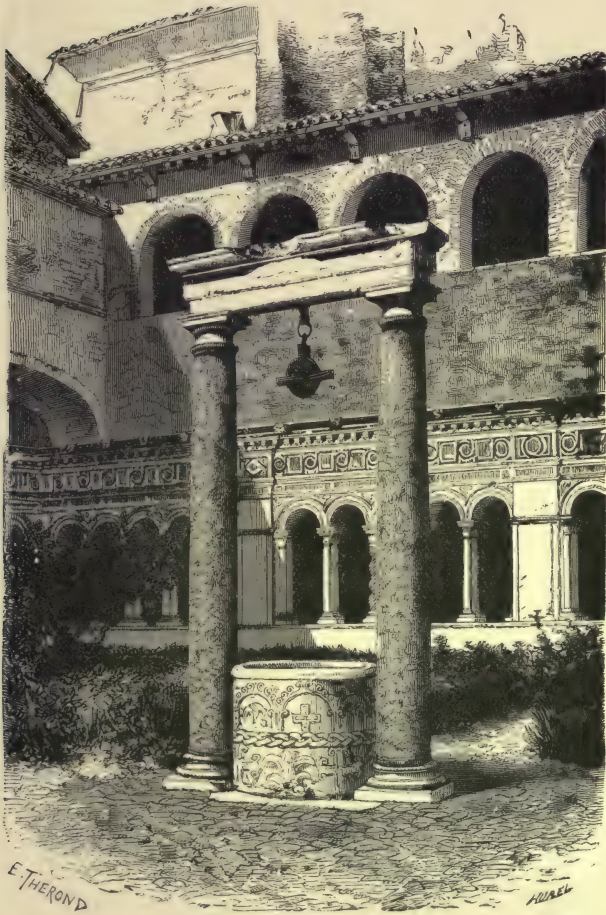
Cloister of St. John Lateran, with Roman Doric Columns. Twelfth Century.
