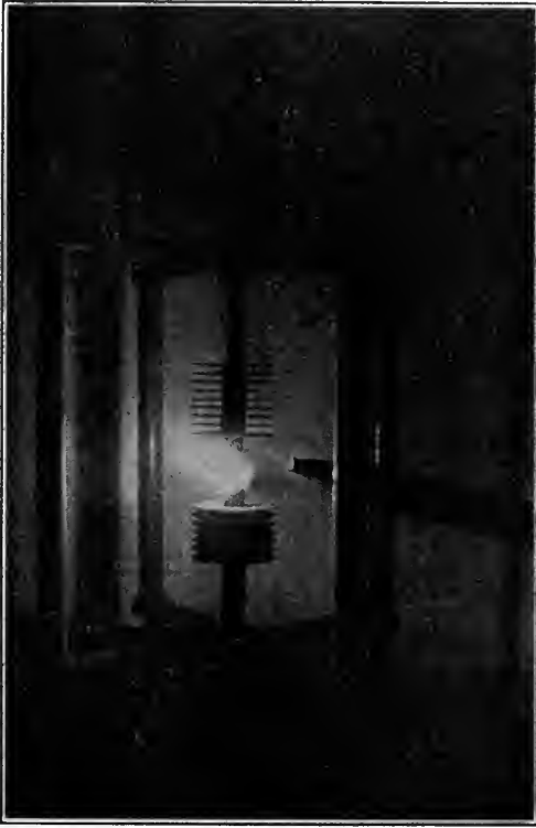
FIG. 4. SPARK GAP OF DE FOREST WIRELESS TRANSMITTING STATION.—By Percival E. Fansler.
