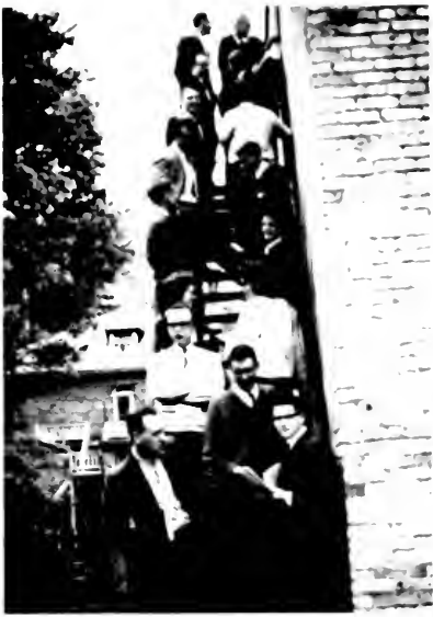
The wrong escape
