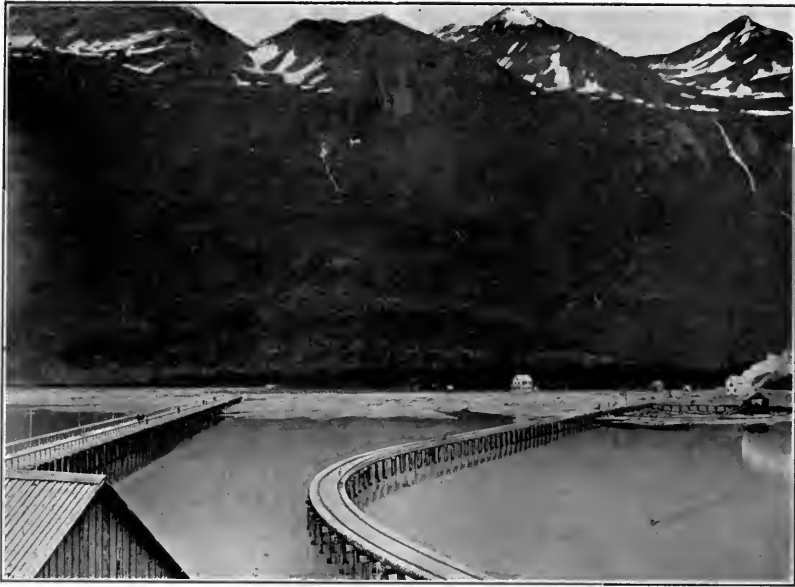
THE RAILWAY PIERS AT VALDEZ
