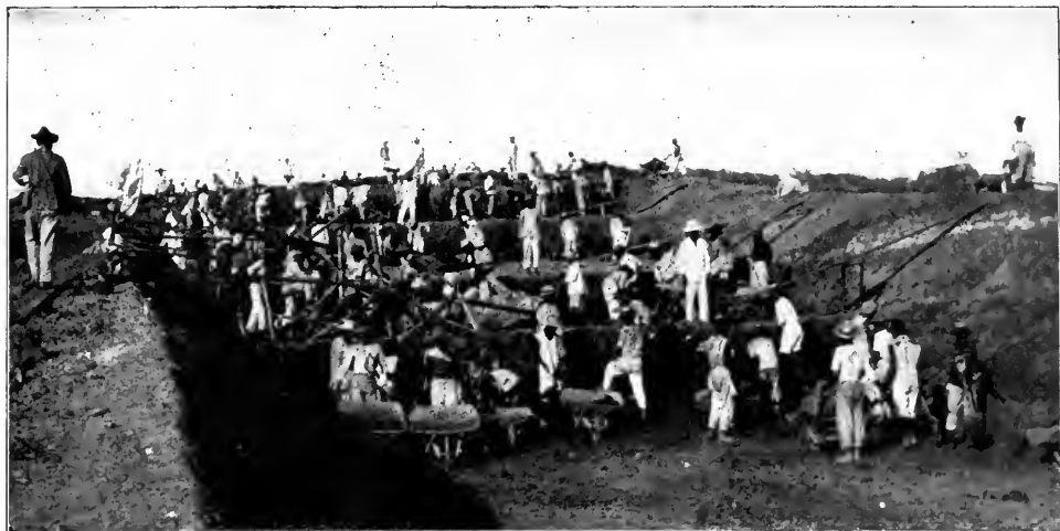
FILIPINOS DIGGING ONE OF THE CUTS FOR THE NEW RAILROAD IN CEBU
