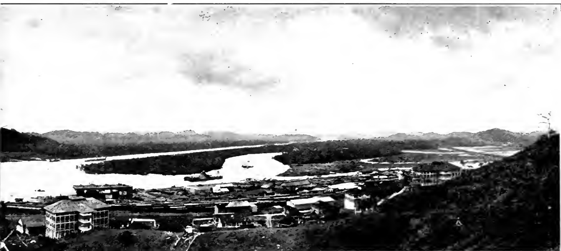
t Pacific terminal of canal. Rio Grande and canal beyond
