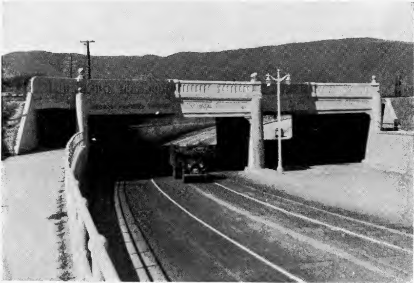
RAILROAD UNDERPASS AT SEATTLE, WASH. OVER 600 RAILWAY CROSSINGS HAVE BEEN ELIMINATED WITH AID FROM THE PWA PROGRAMS
