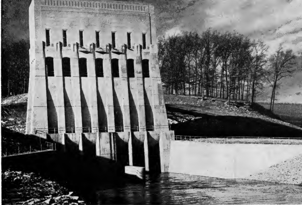
CONTROL GATES ON THE BOLIVAR DAM, ONE OF 14 DAMS CONSTRUCTED IN THE MUSKINGUM VALLEY OF OHIO FOR FLOOD REDUCTION
