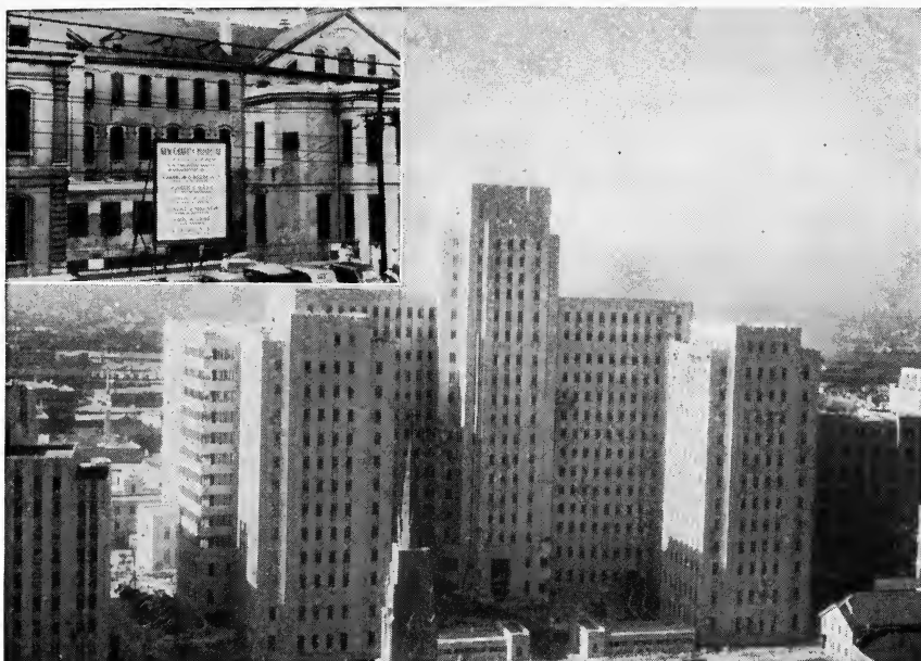
CHARITY HOSPITAL, NEW ORLEANS, THE LARGEST MEDICAL INSTITUTION IN THE SOUTH, WHICH HAS REPLACED THE OLD HOSPITAL SHOWN IN THE INSET
