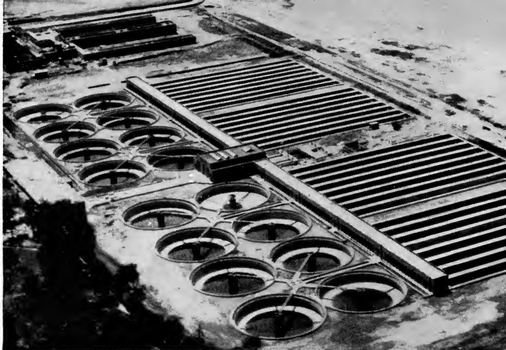
THE EASTERLY SEWAGE-TREATMENT WORKS, PART OF THE VAST SEWAGE-TREATMENT PROGRAM UNDERTAKEN WITH PWA ASSISTANCE IN CLEVELAND, OHIO
