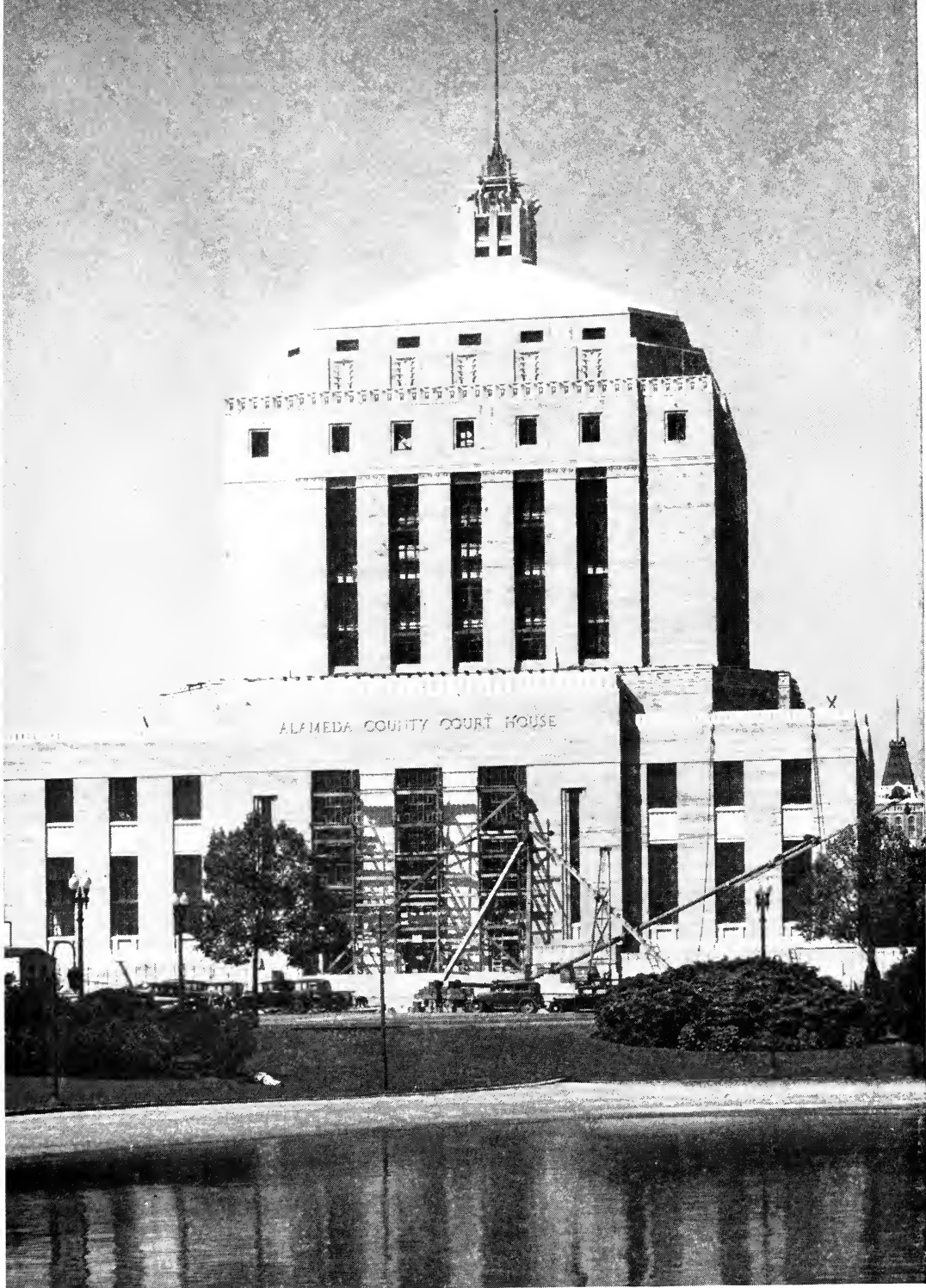
THE NEW ALAMEDA COUNTY COURTHOUSE AT OAKLAND, CALIF., WHICH CONTAINS COUNTY OFFICES, A LAW LIBRARY, AND THE DISTRICT ATTORNEY'S OFFICE AS WELL AS NUMEROUS COURTROOMS. THE STRUCTURE WAS COMPLETED IN 1936
