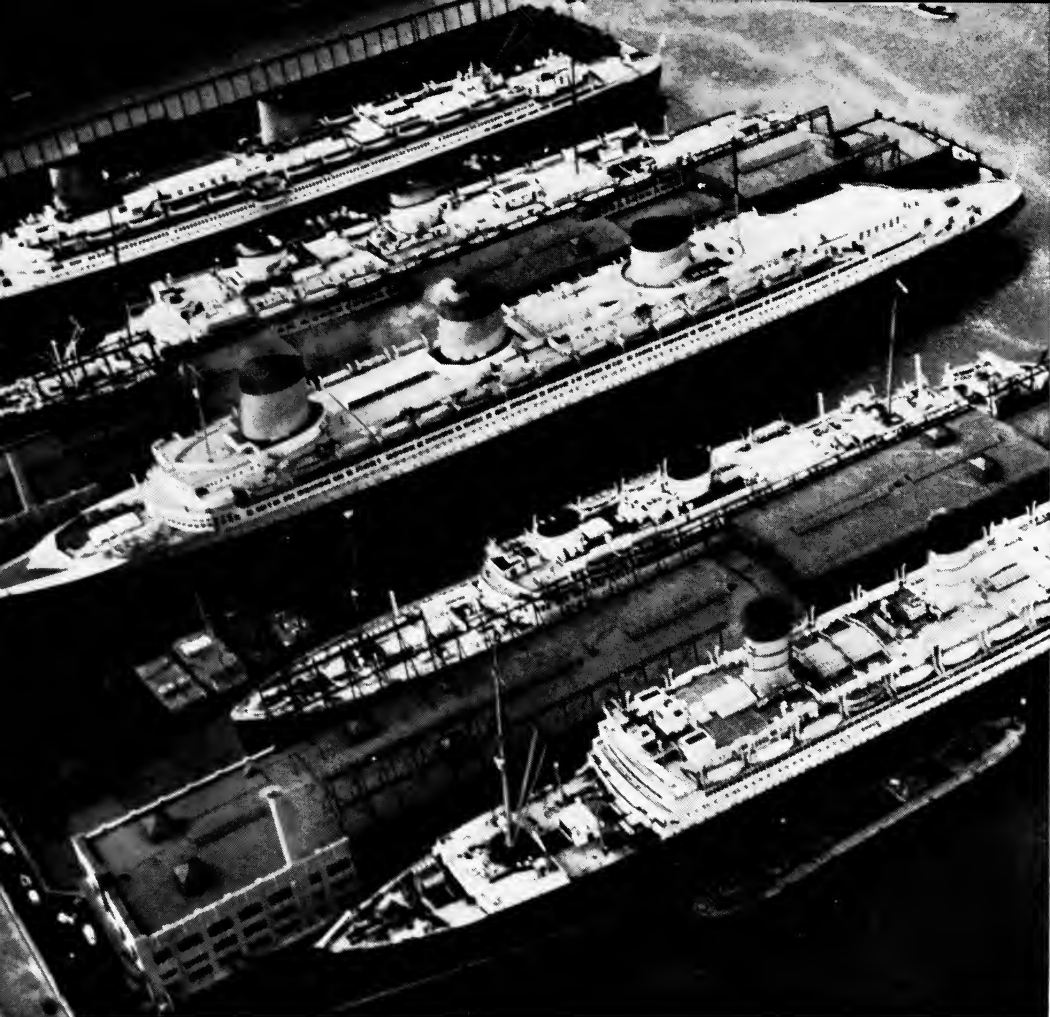
SUPER PIERS FOR SUPER SHIPS. PWA MADE GRANTS TO AID THE CITY OF NEW YORK TO BUILD THREE PIERS COMPRISING THE LARGEST AND MOST MODERN SHIP TERMINAL. DOCKED AT THIS "INTERNATIONAL GRAND CENTRAL STATION" ARE (FROM TOP LEFT TO BOTTOM RIGHT) THE S. S. "EUROPA," "REX," "NORMANDIE," "GEORGIC" AND "BERENGARIA," FIVE OF THE LARGEST SHIPS IN THE WORLD
