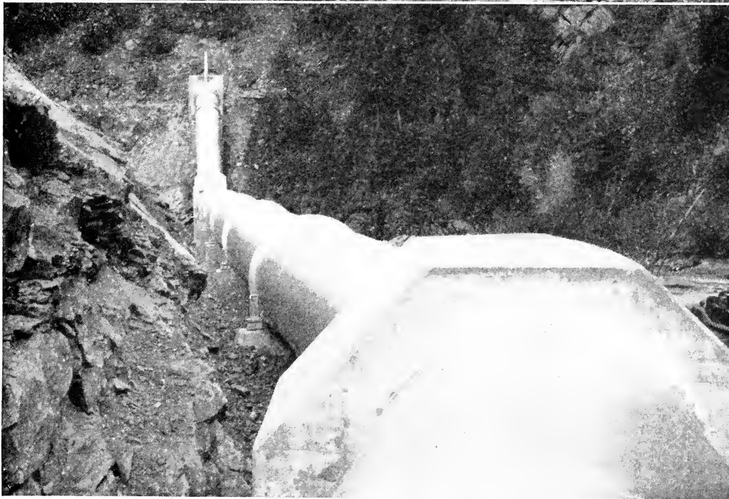
TWO VIEWS OF THE SPECTACULAR DENVER WATER SUPPLY PROJECT, FAMILIARLY KNOWN AS THE MOFFAT TUNNEL PROJECT. UPPER PHOTO SHOWS STILLING BASIN AND CONCRETE-LINED CHUTE AT INTAKE TO RALSTON RESERVOIR. THIS WATER FROM THE WESTERN SLOPE HAS JUST DESCENDED THROUGH A HUGE CONCRETE BOX CHUTE AND IS BEING CALMED IN THE STILLING BASIN BEFORE FLOWING ON TOWARD RALSTON DAM. LOWER PHOTO SHOWS 33-INCH SIPHON NO. 1 IN SOUTH BOULDER CANYON, PART OF THE SOUTH BOULDER DIVERSION CONDUIT
