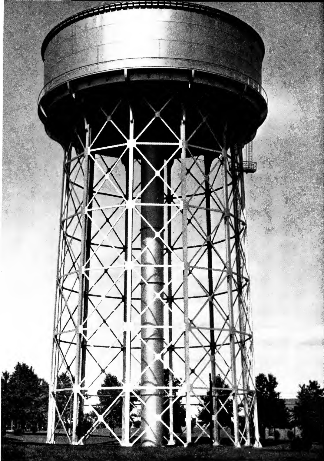
A MILLION-GALLON WATER-STORAGE TANK ERECTED AT NEWPORT NEWS, VA., TO REPLACE AN OLD TANK WHICH HAD BEEN CONDEMNED
