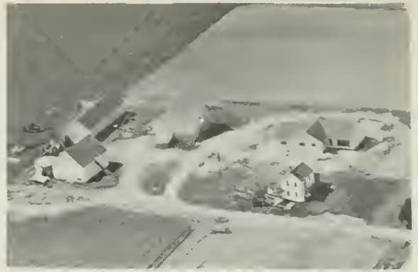
BUTZOW, MARSHALL Rt.1-New home being constructed 120 acres
