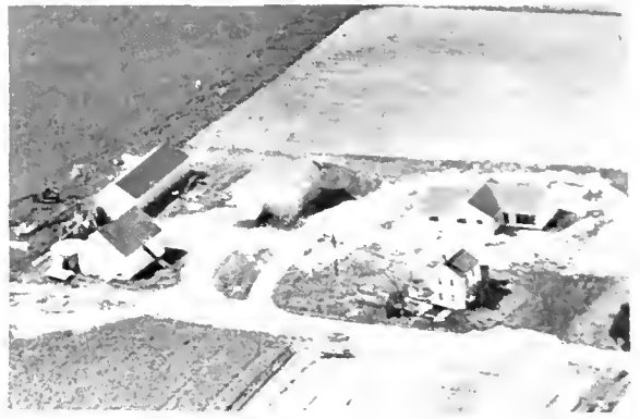
BUTZOW, MARSHALL Rt.1-New home being constructed 120 acres
