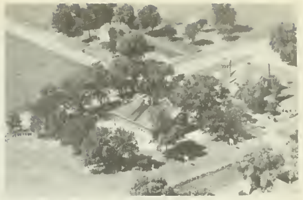
PUBLIC SCHOOL (Built 1912)
