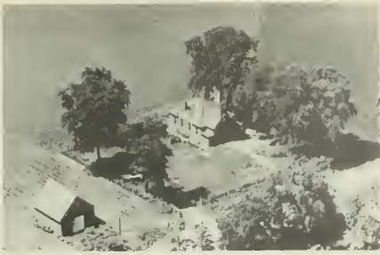
CENTRAL SCHOOL (Built 1897) Rt.1, Fithian
