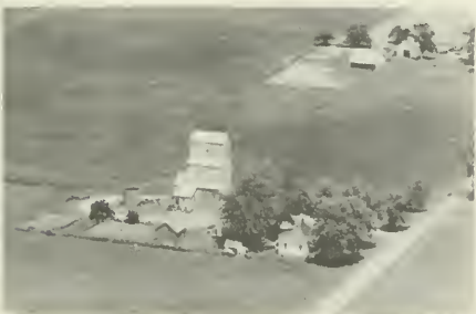
THOMAS, STATION ELEVATOR Rt. 1
