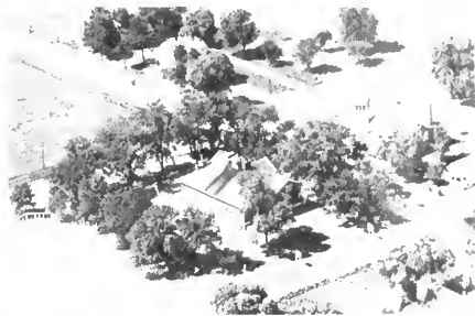
PUBLIC SCHOOL (Built 1912)
