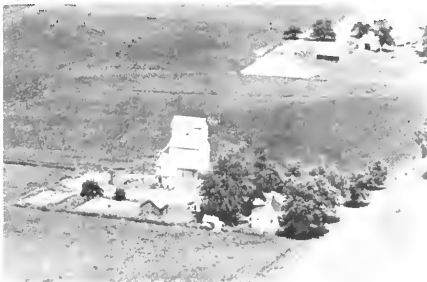
THOMAS, STATION ELEVATOR Rt. 1
