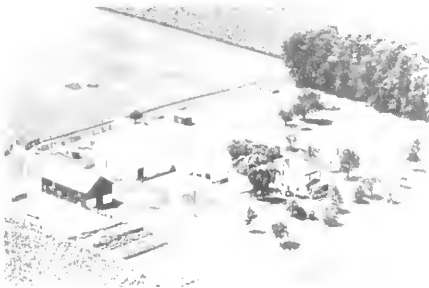
CONDIFF, GUY Rt. 1
