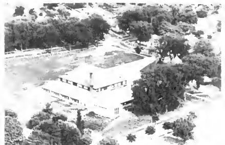
ROSSVILLE COMMUNITY CONSOLIDATED GRADE SCHOOL
