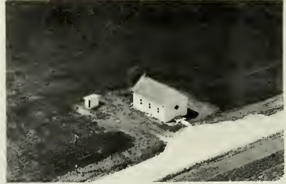
PRAIRIE CREEK TOWN HALL Emden
