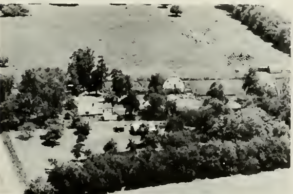
GASAWAY ESTATE Rt. 1 Mt. Pulaski-Geo. Wilham, Opr.
