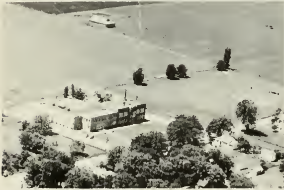
HARTSBURG-EMDEN SCHOOL Dist. 21 Hartsburg
