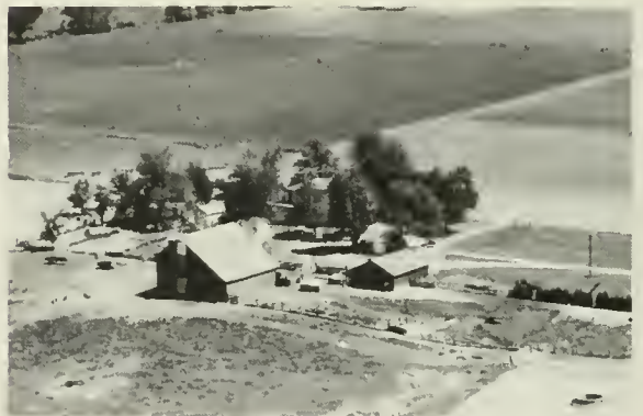
FITZSIMONS, HAZARD Rt. 1
