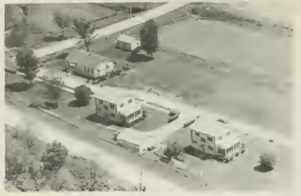
FIELD HOUSE New LaGrange Lock Versailles Daniel A. Ballard (Center) Walter Carlock
