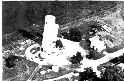
FERRIS ELEVATOR CO. Ferris
