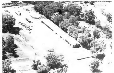
HANCOCK COUNTY HIGHWAY DEPARTMENT Carthage
