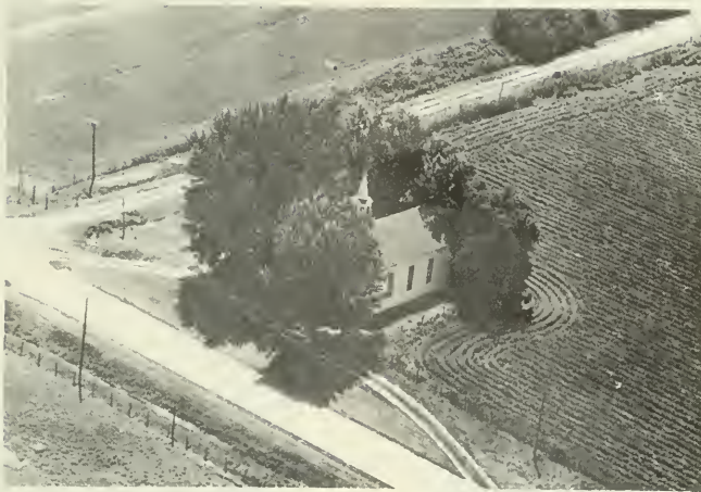
CENTER PRAIRIE METHODIST CHURCH Sec. 26 Williamsfield
