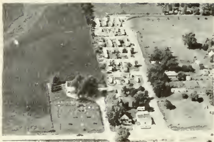
WEST MAIN TRAILER COURT 1719 West Main Galesburg Sec. 9
