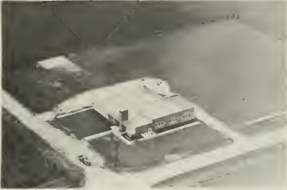
BURNS SCHOOL UNIT # 224 Galva Built 1951
