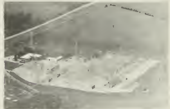
KEWANEE SUB STATION (Electricity) Kewanee Rt. 3
