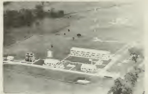
NATURAL GAS COMPRESSOR STATION New Windsor 80 acres
