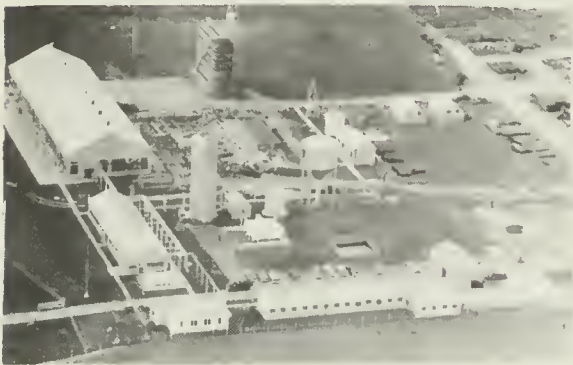
NATURAL GAS PIPELINE CO. OF AMERICA Geneseo Est. 1930 30 acres A. Yingling Supt.
