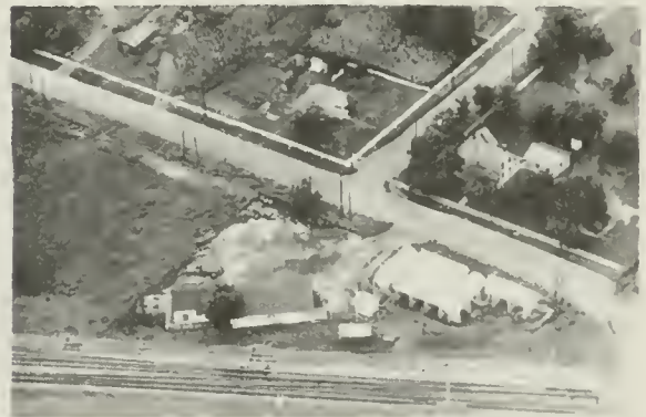
STANDARD OIL CO. (BULK PLANT) Kewanee D. Fisher Agent 1123 New St.
