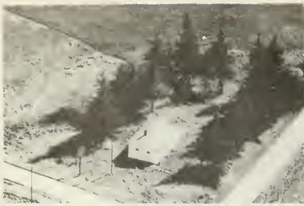
CENTRAL SCHOOL Sec. 36 Rt. 1 West Point Discontinued 1951
