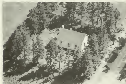
CHRISTIAN HALL COMMUNITY HOUSE Winslow Rt. 1
