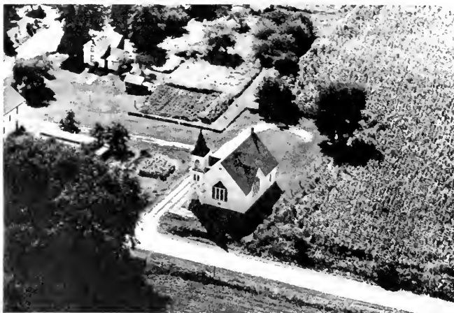
GRACE CHURCH Erected 1895
