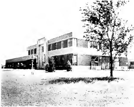
DISTRICT NO. 4 Office and Garage Building, Peoria.
