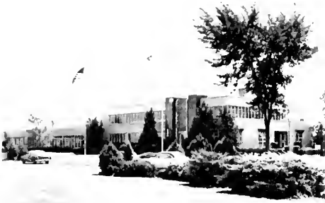
DISTRICT NO. 9 Office and Garage Building, Carbondale.
