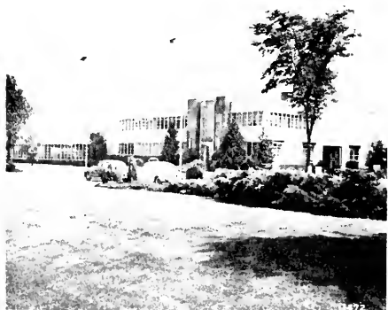
DISTRICT NO. 9 Office and Garage Building, Carbondale.
