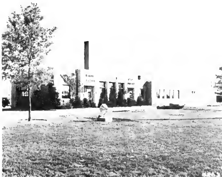
STATE HIGHWAY POLICE DISTRICT HEADQUARTERS Station located 5 miles south of Effingham on U.S. Route 45.
