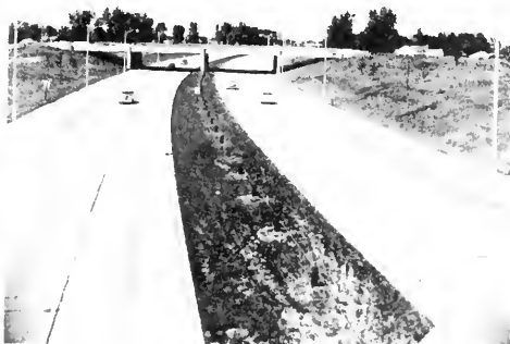
Grade Separation on Edens Expressway in Morton Grove, Cook County.
