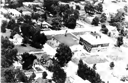
PRINCEVILLE COMMUNITY CONSOLIDATED PRINCEVILLE GRADE SCHOOL
