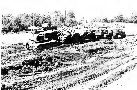
Heavy grading equipment, south of Mt. Sterling, Brown County.
