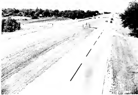
Typical modernization of pavement, U. S. Route 66 at Farmersville, Montgomery County.
