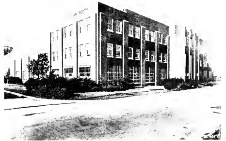
DISTRICT NO. 6 Office and Garage Building Springfield.
