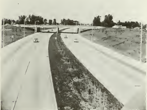
Grade Separation on Edens Expressway in Morton Grove, Cook County.
