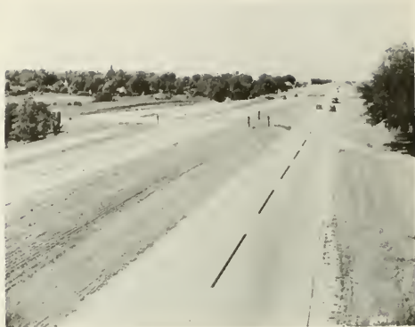
Typical modernization of pavement, U. S. Route 66 at Farmersville, Montgomery County.
