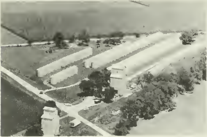
QUAKER OATS ELEVATOR RISK STATION Strawn
