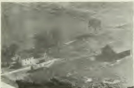
BEAMAN LOUIS ESTATE Rt. 1 Manville Mgr. Cashmer, Clifford C. Tenant House
