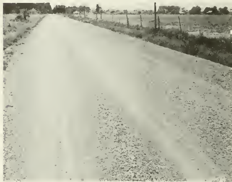
Typical Farm to Market Township Road, Ob-long Township, Crawford County.
