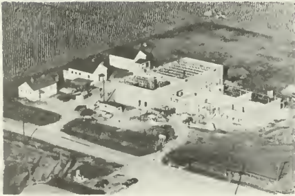
OMEGA ELEMENTARY CONSTRUCTION SCHOOL Pontiac Rt. 6 2 acres
