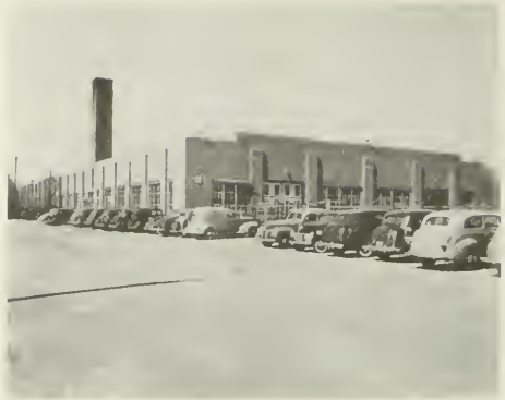
CENTRAL GARAGE State Highway Central Gar- rage Building, Springfield.
