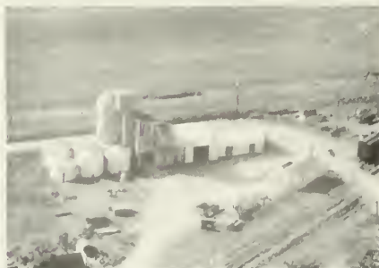
JACOBSON GRAIN ELEVATORS Rowe, Illinois
