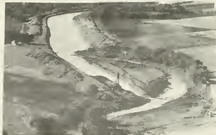
STRAIGHTENING & WIDENING THE VERMILION RIVER CHANNEL November 1954 Between Pontiac & Fairbury
