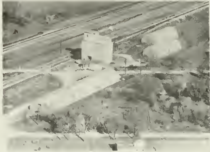
JACOBSON GRAIN ELEVATORS Cayuga, Illinois
