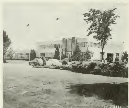
DISTRICT NO. 9 Office and Garage Building, Carbondale.
