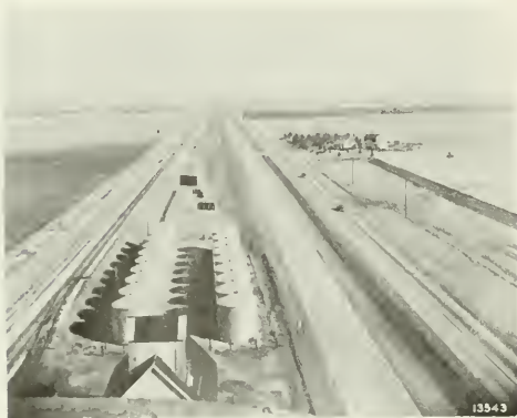
Typical modernization of pavement, U.S. Route 66 north of Lincoln, Logan County.
