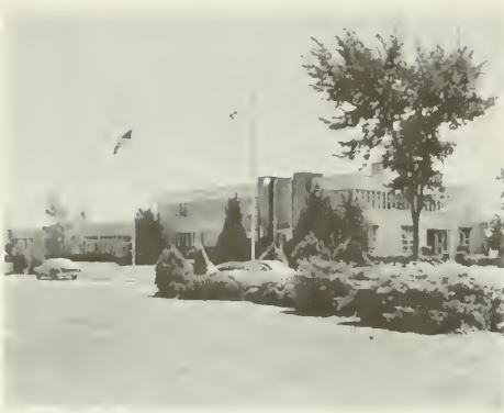
DISTRICT NO. 9 Office and Garage Building, Carbondale.
