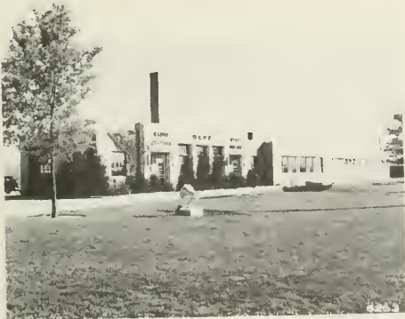
STATE HIGHWAY POLICE DISTRICT HEADQUARTERS Station located 5 miles south of Effingham on U.S. Route 45.
