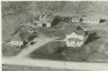
LARSON AUGUST W. Cornell Gas Well On Farm
