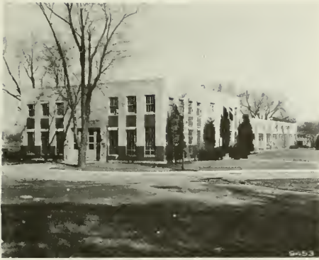
DISTRICT NO. 2 Office and Garage Building, Dixon.
