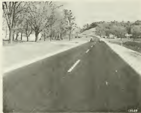
Bituminous surfaced pavement, U.S. Route 36 near Winchester, Scott County.
