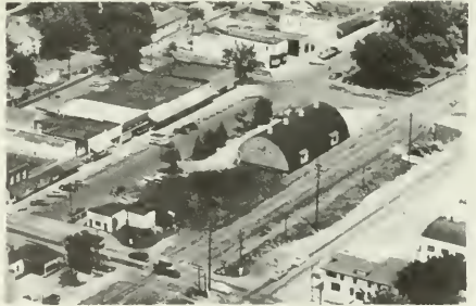
LIVINGSTON GRAIN & SUPPLY WAREHOUSE Chatsworth
