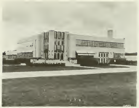
DISTRICT NO. 3 Office and Garage Building, Ottawa.
