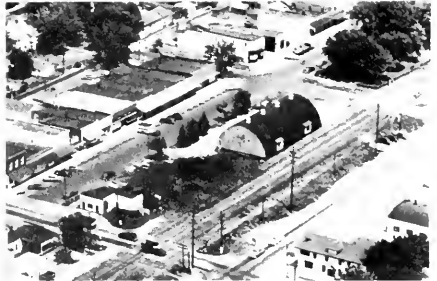
LIVINGSTON GRAIN & SUPPLY WAREHOUSE Chatsworth
