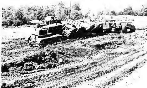
Heavy grading equipment, south of Mt. Sterling, Brown County.
