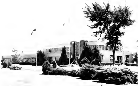
DISTRICT NO. 9 Office and Garage Building, Carbondale.
