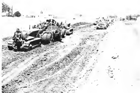
Heavy grading equipment making grade change, U.S. Route 51 north of Vandalia, Fayette County.
