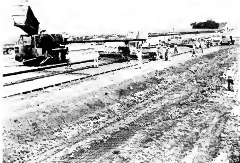
Typical paving operation, U. S. Route 66, north of Williamsville, Sangamon County.
