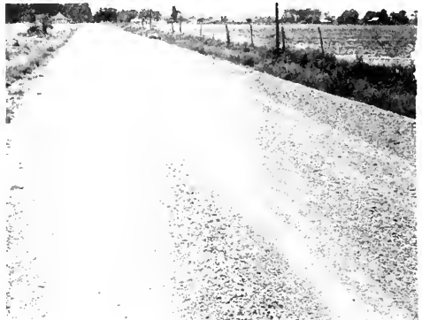
Typical Farm to Market Township Road, Ob-long Township, Crawford County.
