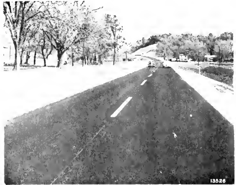
Bituminous surfaced pavement, U.S. Route 36 near Winchester, Scott County.
