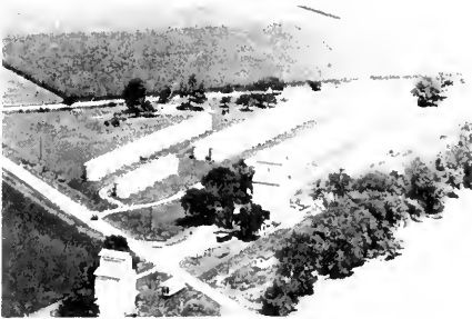
QUAKER OATS ELEVATOR RISK STATION Strawn
