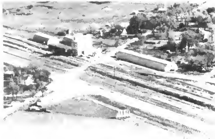
JACOBSON GRAIN ELEVATOR Cayuga
