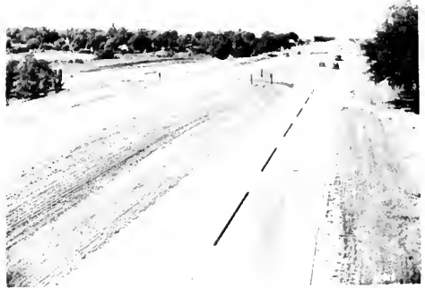
Typical modernization of pavement, U. S. Route 66 at Farmersville, Montgomery County.
