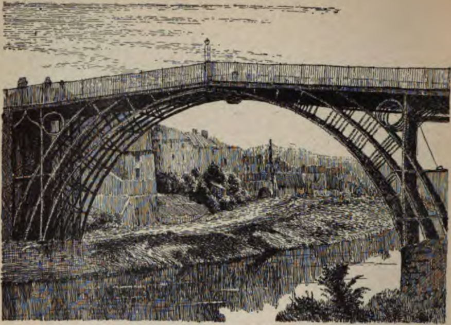
FIRST IRON RAILROAD BRIDGE IN ENGLAND.
