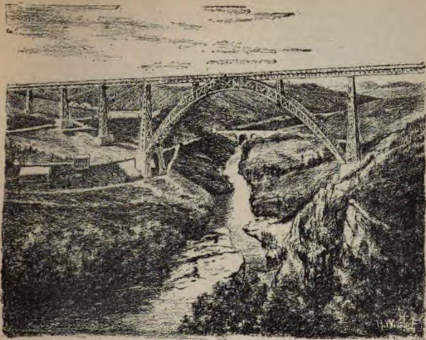
THE HIGHEST IRON ARCH IN THE WORLD,
