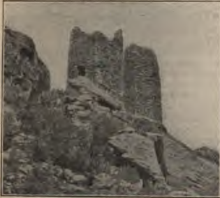
TWIN TOWER IN RUIN CANYON.
