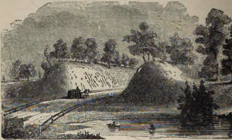
GRADED ROAD IN OHIO.
