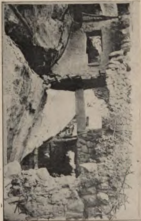
PLASTERED PILLAR IN CLIFF PALACE.
