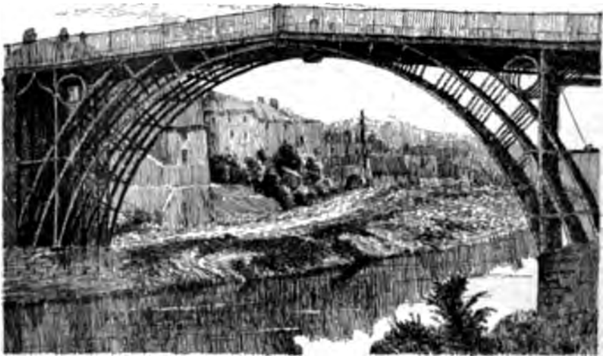
BRIDGE ON FALLOOY FIDGE IN ENGLAND
