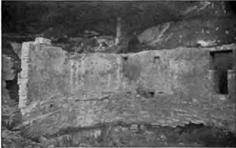
INTERIOR OF CIRCULAR ROOM (Mancos Canon.
