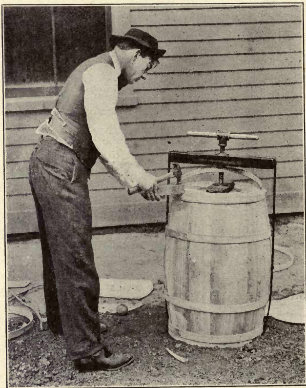
HEADING UP THE BARREL—SCREW PRESS
