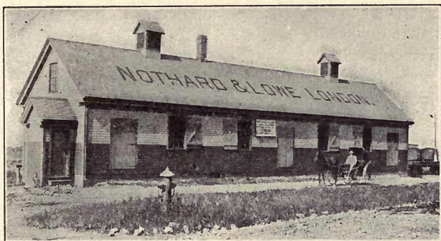
A COMMERCIAL VENTILATED STORAGE HOUSE IN NOVA SCOTIA
