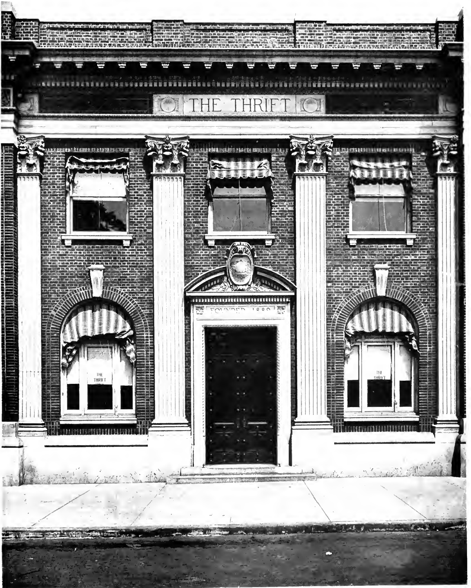
ENTRANCE DETAIL, THE THRIFT BANK, DE KALB AVENUE CORNER RYERSON STREET, BROOKLYN, N. Y. Shampan & Shampan, Architects.
