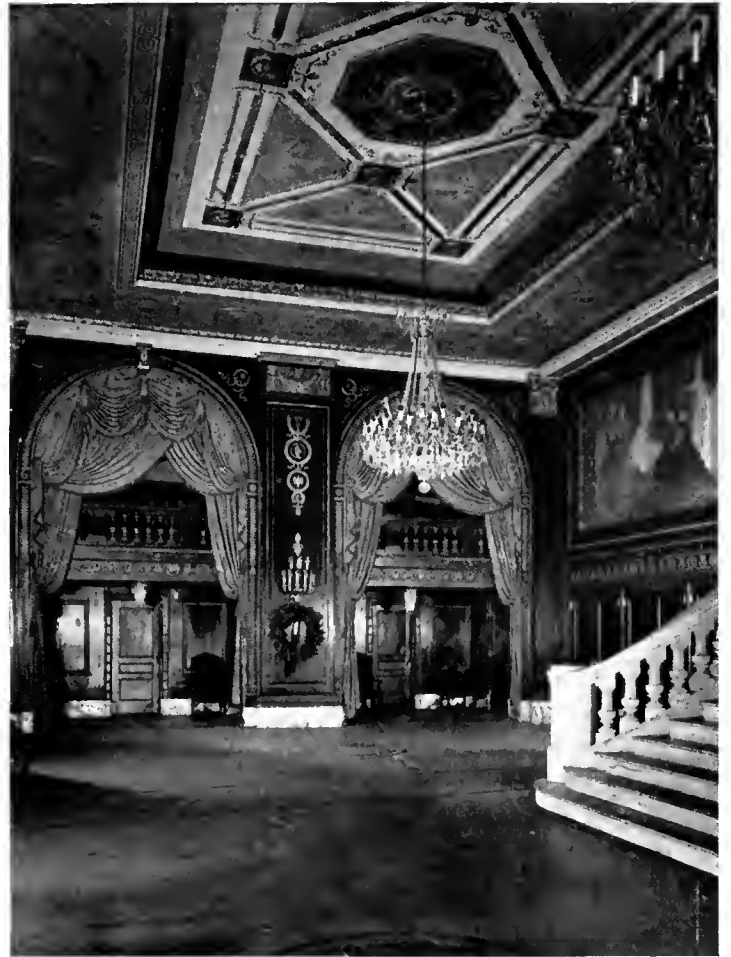
Grand lobby and part of main staircase, Capitol Theatre, New York. Thos. W. Lamb, Architect.
