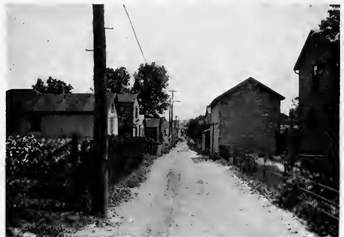
Alley housing, Dayton, Ohio.
