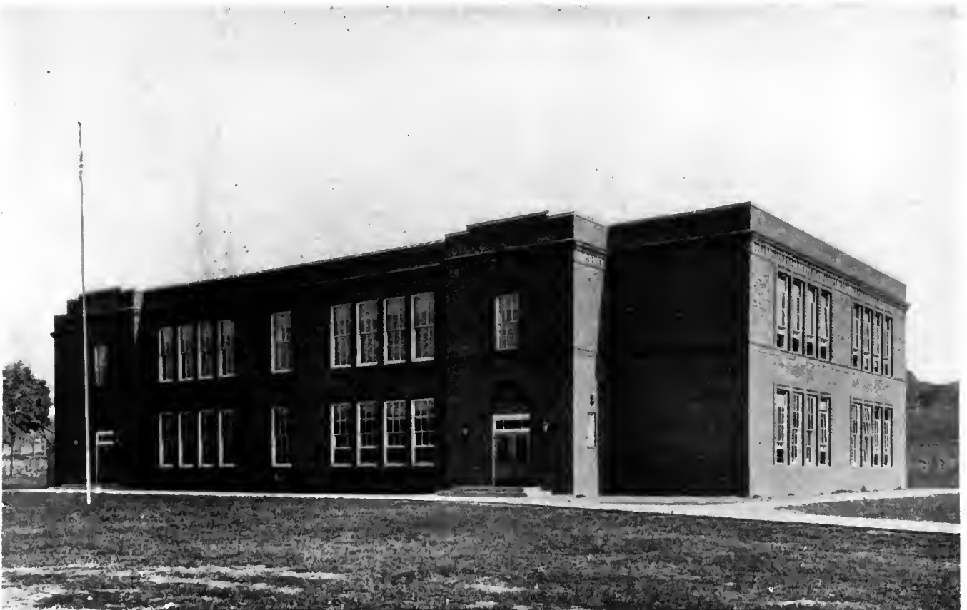
FERRIS AVENUE GRADE SCHOOL, WHITE PLAINS, N. Y. Tooker & Marsh, Architects. Arthur W. Coote, Associate. TWO TYPES OF SCHOOL OF ALL BRICK DESIGN (RECENTLY COMPLETED).
