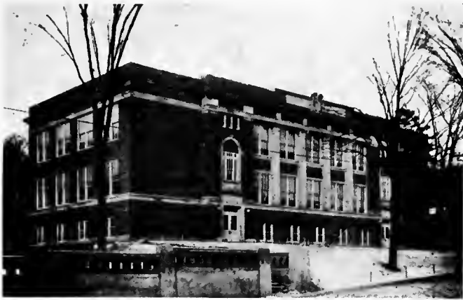
Combination grade and high school, Port Henry, N. Y. Tooker & Marsh Architects. Arthur W. Coote, Associate.
