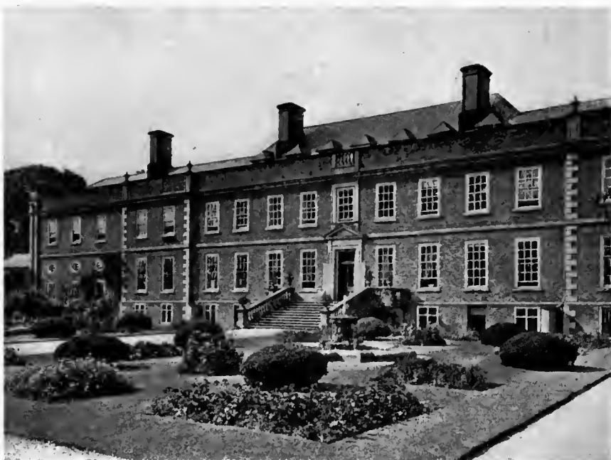
Erddig Park, Derbyshire.
