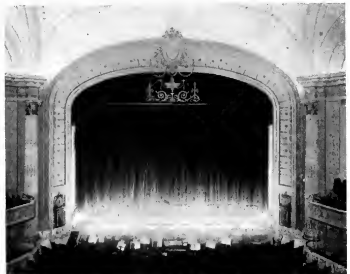
Detail looking toward stage, showing effect of cove footlights. Theatre in Brooklyn, N. Y. Thos. W. Lamb, Architect.
