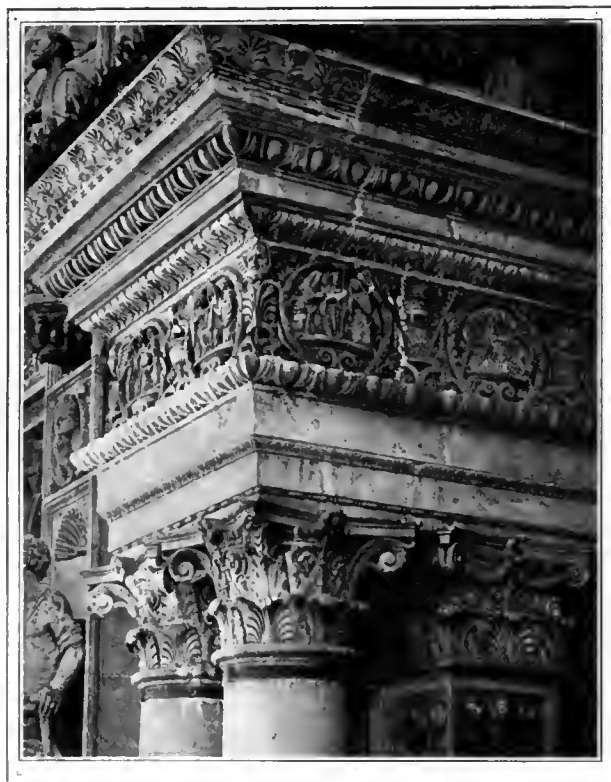
The façade—capitals with entablature and cornice.
