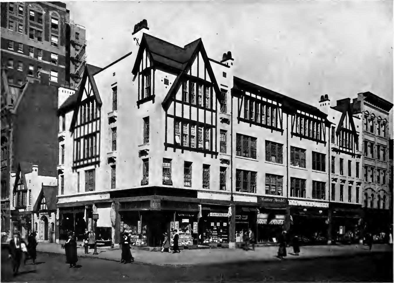
Remodelled shops and apartments corner Broadway and 80th Street, New York. B. H. & C. N. Whinston, Architects.
