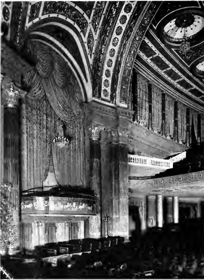
Sounding board and proscenium treatment, also showing balcony side walls, Capitol Theatre, New York. Thos. W. Lamb, Architect.
