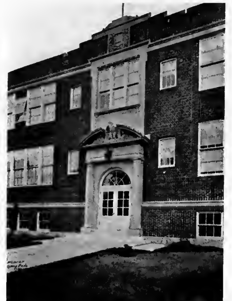
Entrance detail, school, Glens Falls, N. Y. Tooker & Marsh, Architects. Arthur W. Coote, Associate.
