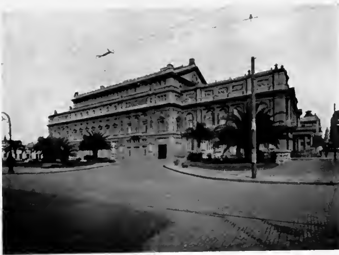
COLON THEATRE. (The exterior of the building shows three different styles of decoration: the first floor in the Ionic style; the second Corinthian; and the third Attic, inclining toward the Corinthian. The height of the façades, from the ground up to the cornice, is 24.70 metres. The playhouse is one of the largest in the world. Its total length from one of the balconies is 75 metres, three metres longer than that of San Carlo in Naples. The dimensions of the ground floor are 27.8 metres by 22.50 metres. It contains 900 fauteuils placed on seven grades. The hall can hold 3,750 spectators. The front of the stage is 18 metres broad by 19.25 metres high. The interior vertical dimension of the stage is 48 metres from the foundations up to the arch. The theatre is constructed with incombustible materials.)
