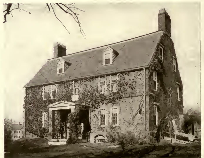
X. Craddock House, present condition.
