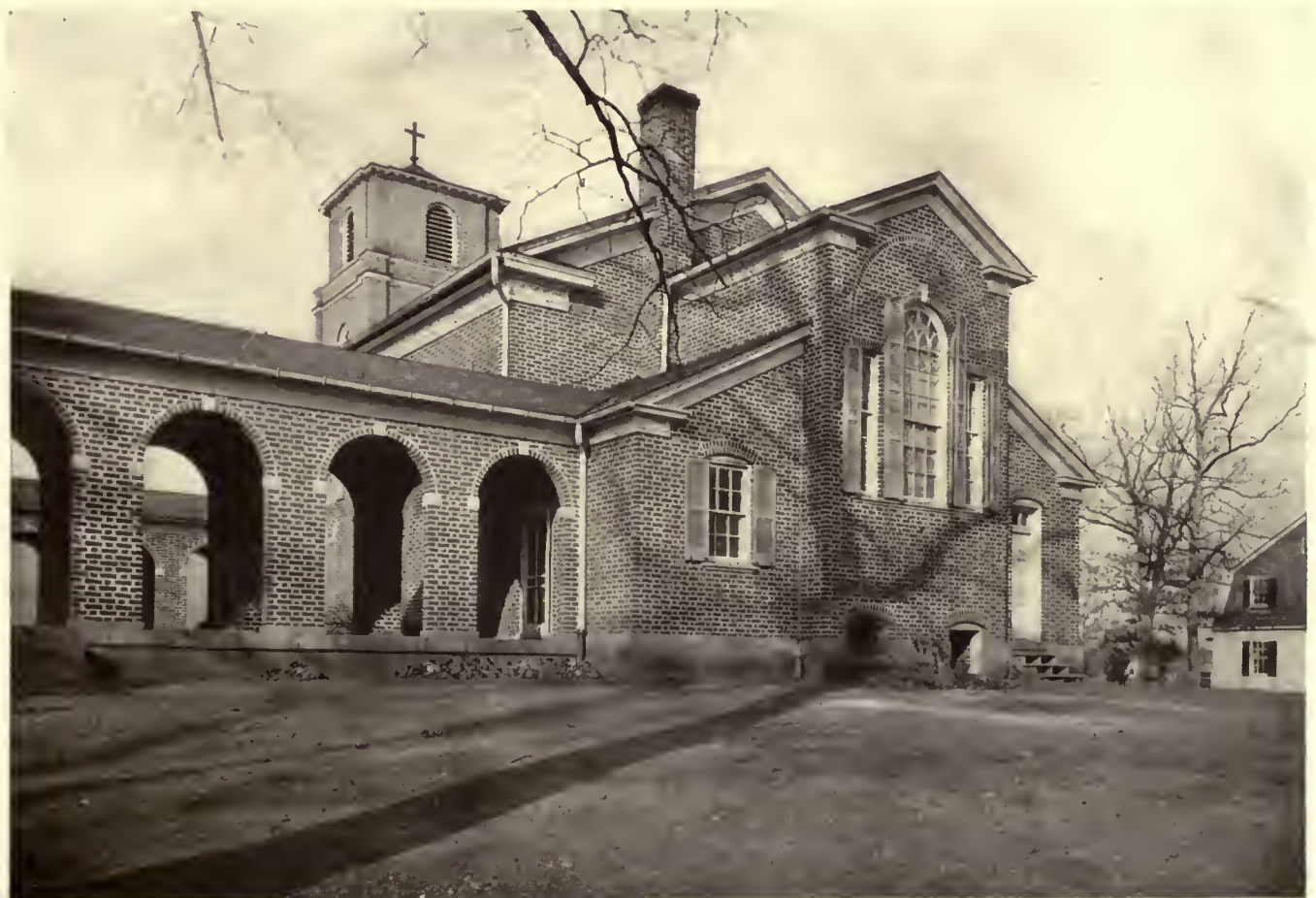
EMANUEL EPISCOPAL CHURCH, GREENWOOD, VA.
