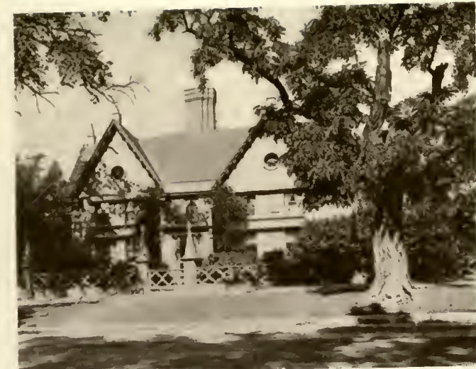
Pickering House, Salem. (Present condition.)
