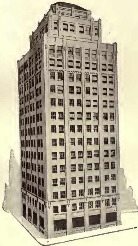
Barrett Specification 20-year Bonded Roof on Hide & Leather Realty Co. building, New York City. Eng. & Gen'l. Cont.: Thompson & Binger, New York; Roofer: New York Roofing Co., New York City.
