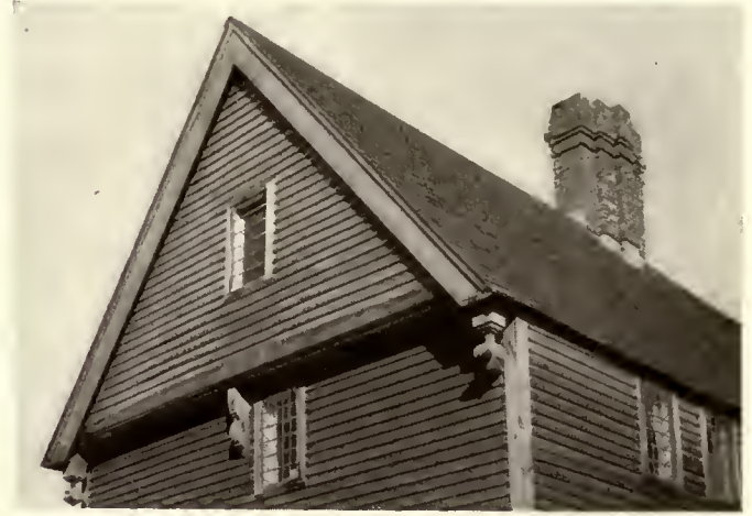
Overhanging gable end with chamfered end girt, bracket and drops; moulded verge board.
