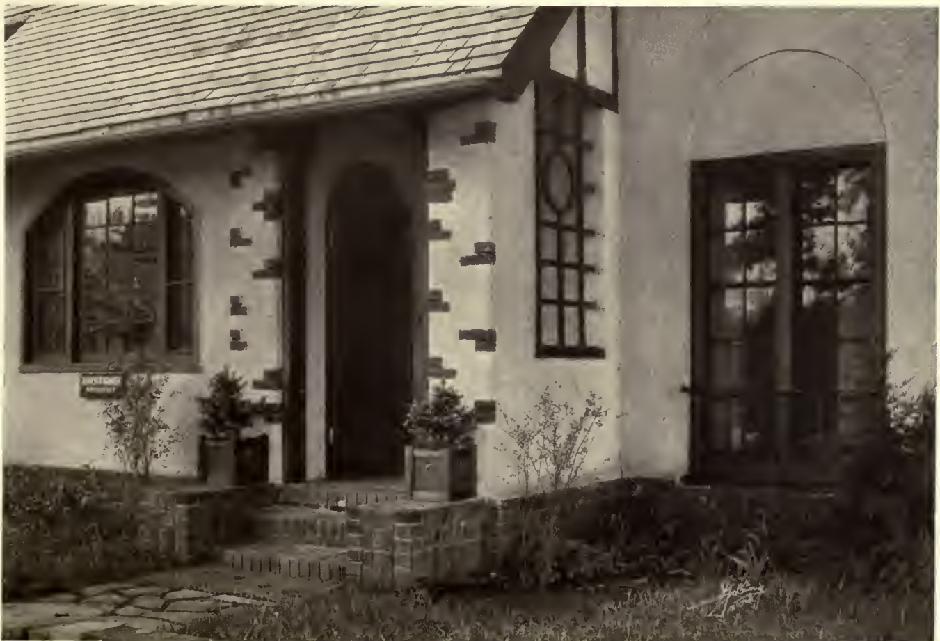
DETAIL OF ENTRANCE.
