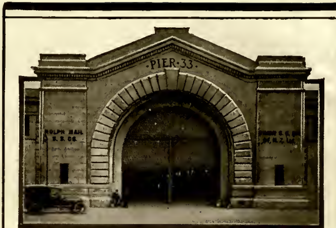
Main Entrance Doors, Pier 33, San Francisco
