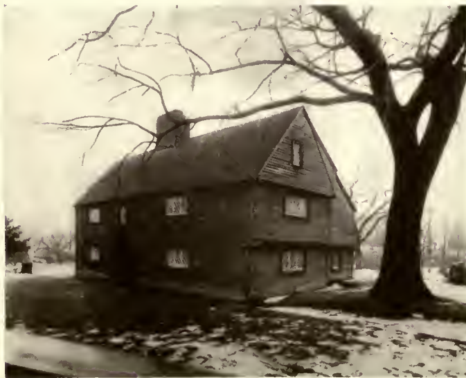
III. Whipple House, Ipswich, with end overhang ("Hewn overhang"), beautifully moulded. Ink line indicates original silhouette.
