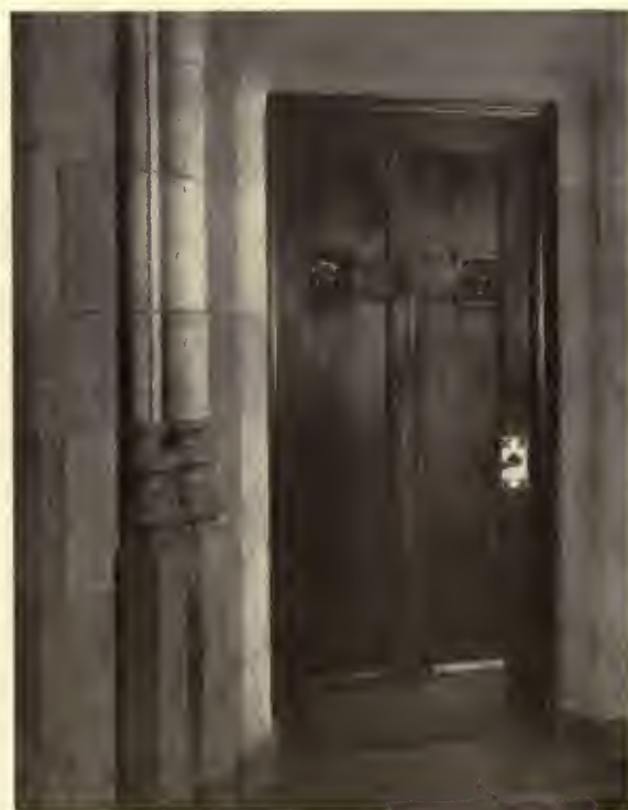
Door detail, main church auditorium.
