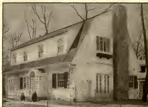
Walls finished with Cabot's Old Virginia White. Roof stained with Cabot's Creosote Stains. F. A. Cooper & Co., Architects, Chicago
