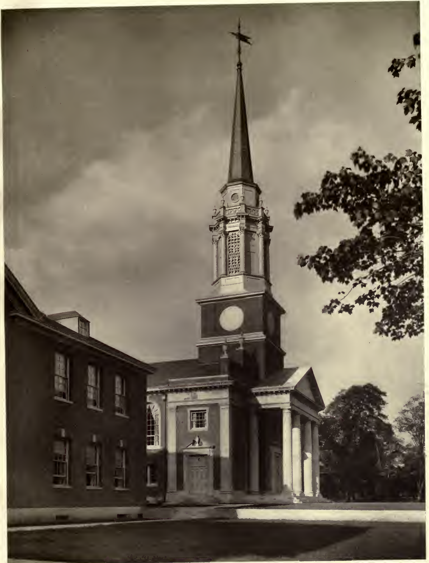
CENTRAL PRESBYTERIAN CHURCH, MONTCLAIR, N. J. Carrère and Hastings, Architects. Shreve, Lamb and Blake, Associated.
