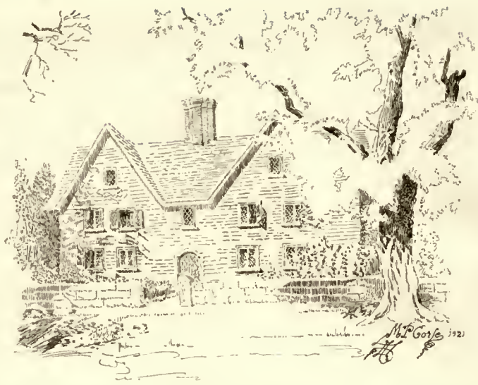
Imaginary restoration, as it may have appeared originally. Drawn directly from photo. Characterless ornament and projecting porch dropped; window-sills raised a few inches; leaded casements substituted for later type; otherwise no alteration has been made in either proportion or detail.
