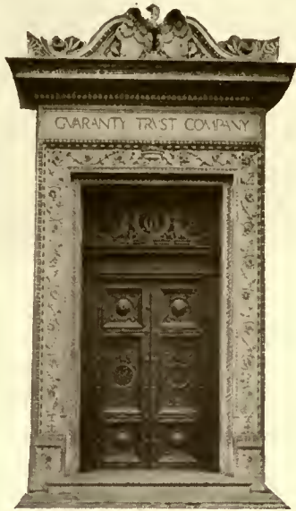
Flanking the entrance of the Guaranty Trust Company's Fifth Avenue offices are exquisite examples of granite carving. York & Sawyer, Architects.
