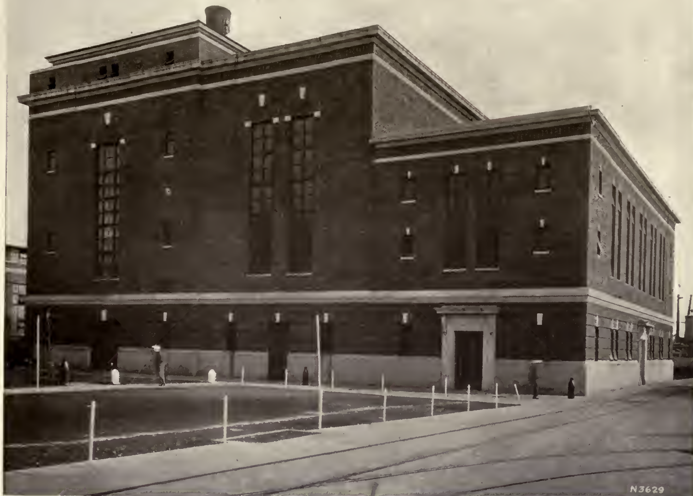
Power-House, Naval Torpedo-Station, Newport, R. I.
