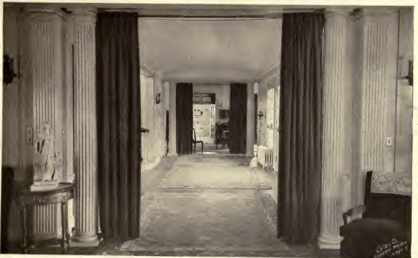
VIEW THROUGH FIRST FLOOR.
