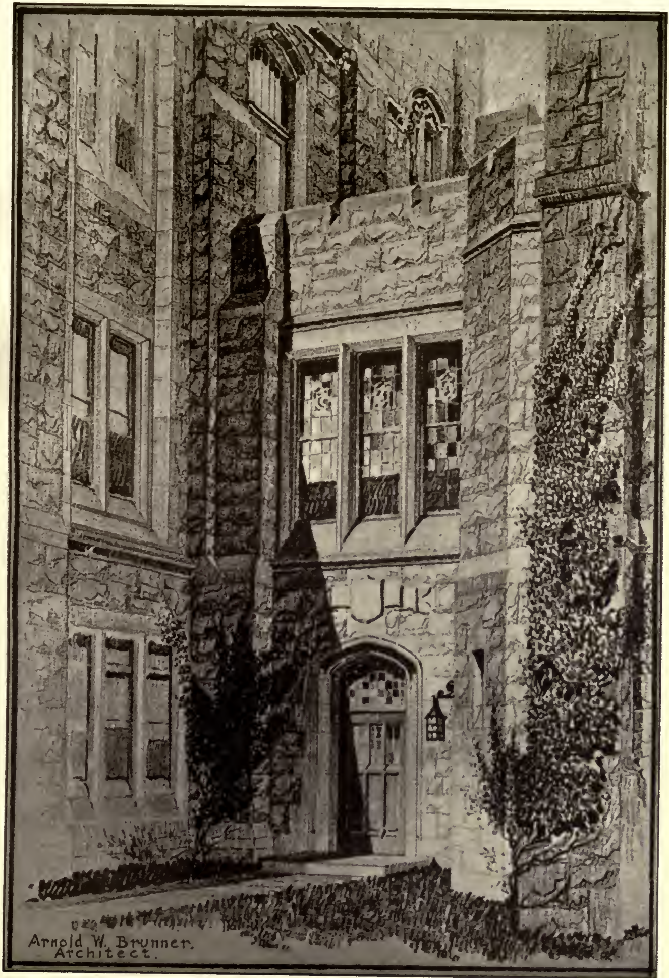
CORRIDOR CONNECTING NEW HOSPITAL WITH PRESENT BUILDING.
