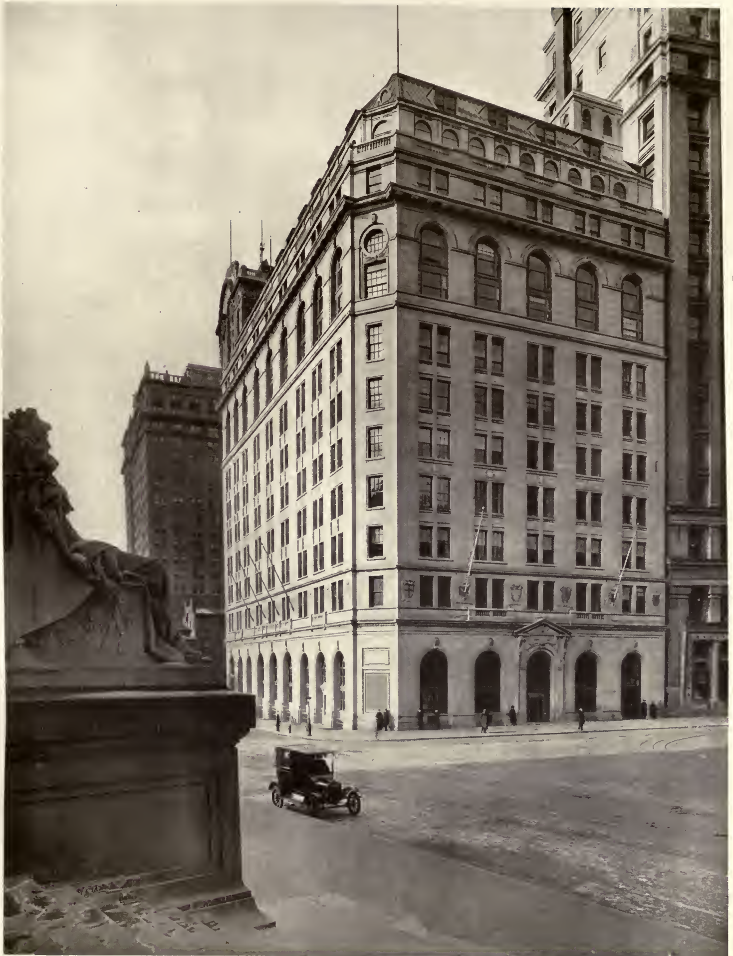
INTERNATIONAL MERCANTILE MARINE BUILDING, No. 1 BROADWAY, NEW YORK.
