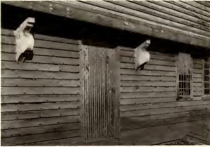
Capen House, Topsfield, near the "Green," restored. Pronounced overhang, with brackets, casement windows (said to be exact size of originals) with rectangular panes, nail-studded.
