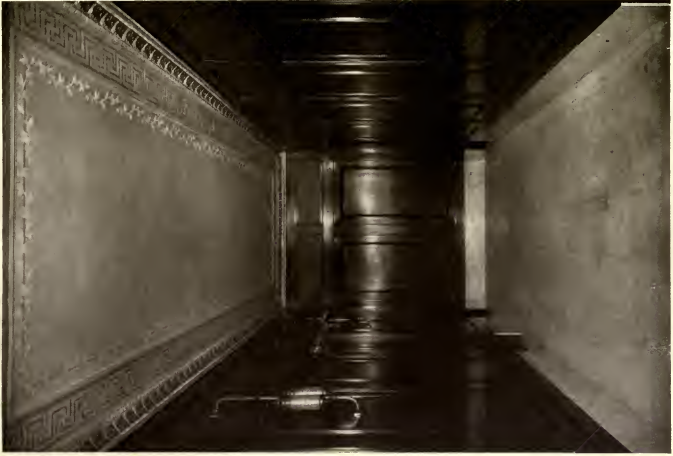
CORRIDOR LEADING TO EXECUTIVE OFFICES FROM MAIN ENTRANCE LOBBY.
