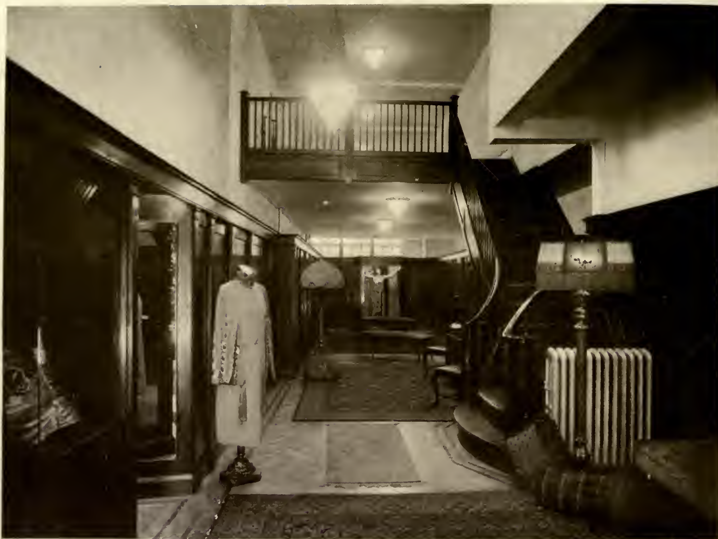
STORE, FIRST FLOOR.
