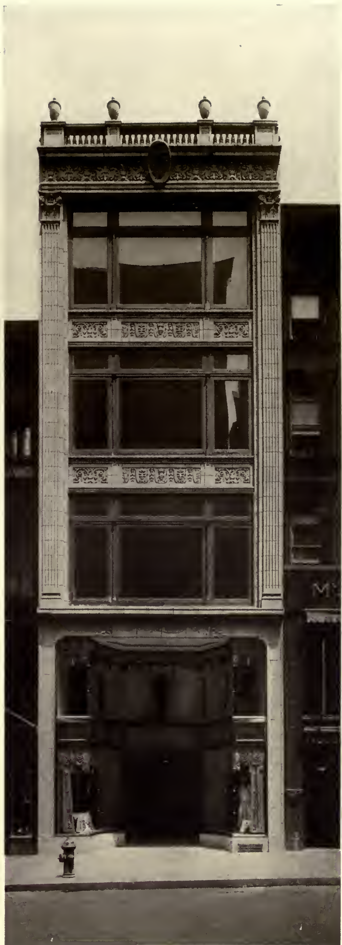
New business building, 131 West 45th Street, New York.
