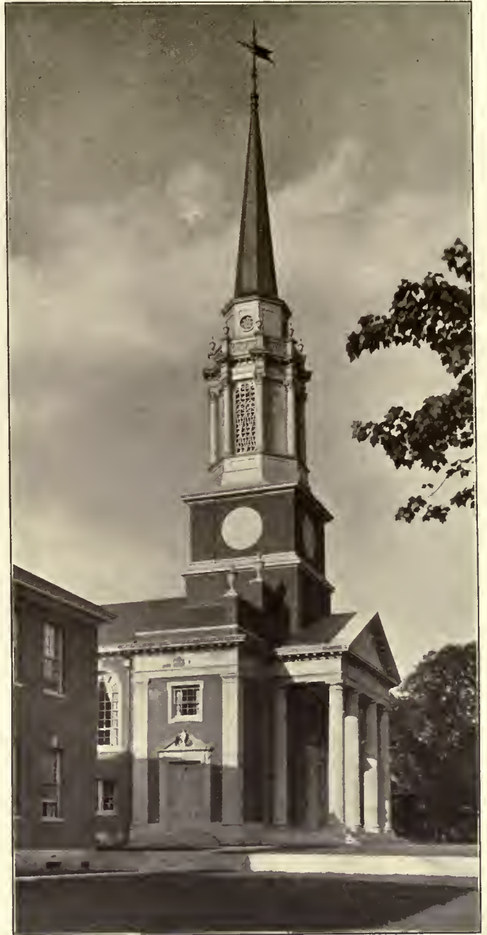
Central Presbyterian Church, Montclair, N. J. Carrère & Hastings, Architects Shreve, Lamb & Blake, Associated
