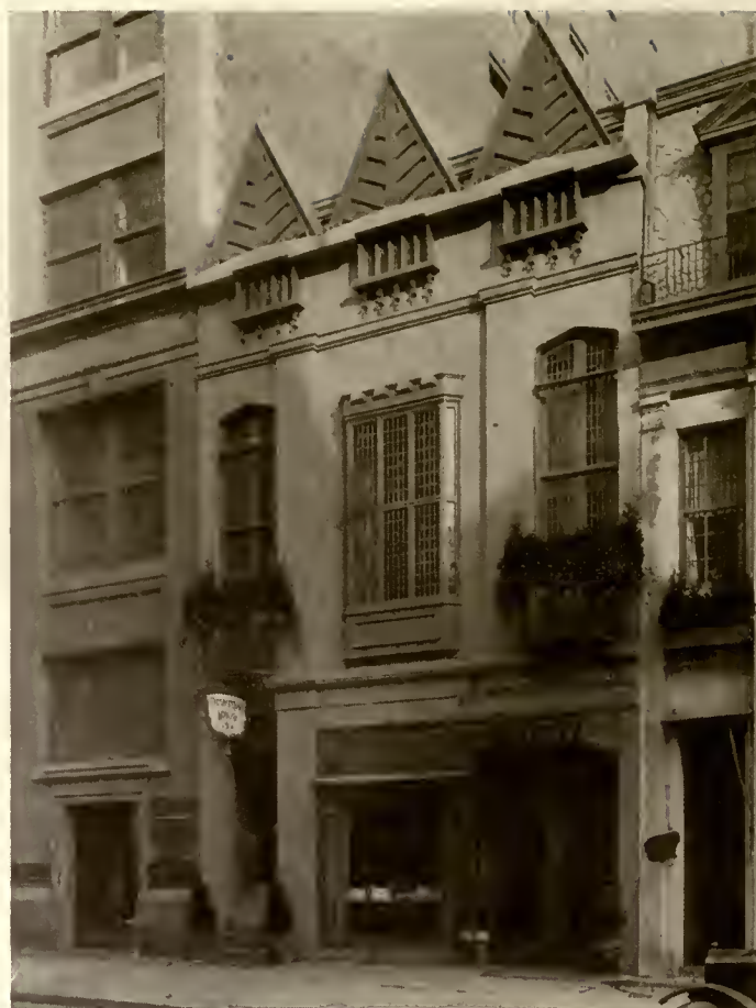
Primrose house, East 52d St., New York. Ekin Wallick, architect.
