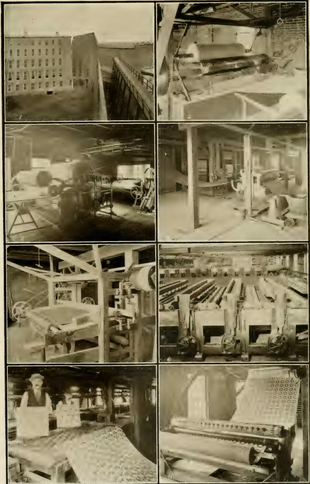
1. Fire Wall and Railroads. 2. Sizing Machine. 3. Calender End of the Sizing Machine. 4. Painting Machine and Drying Racks.
