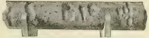
Electrolytically Pitted Water Pipe.
