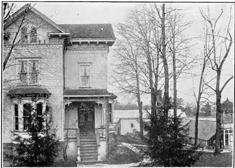
PARTIAL VIEW OF THE LAMBORN GREENHOUSES.
