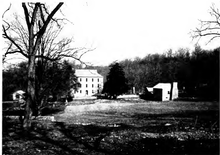
Restored Grist-mill, Spring Mill State Park, Indiana
