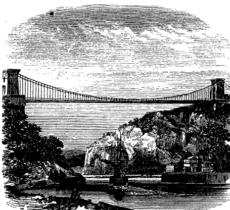
Clifton Suspension Bridge.
