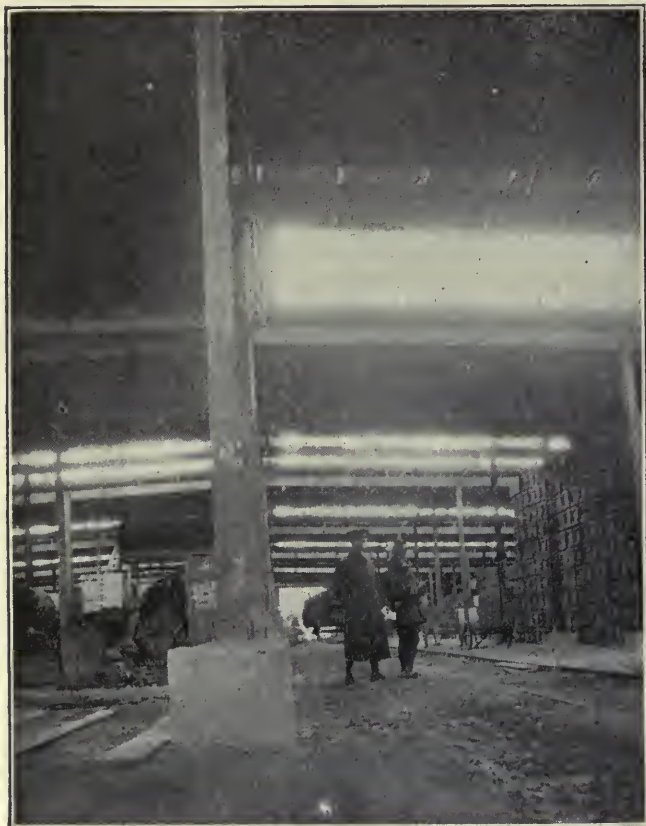
F. WIRE GLASS REPLACES CHEESECLOTH IN THE ORDNANCE BUILDING MONITORS
