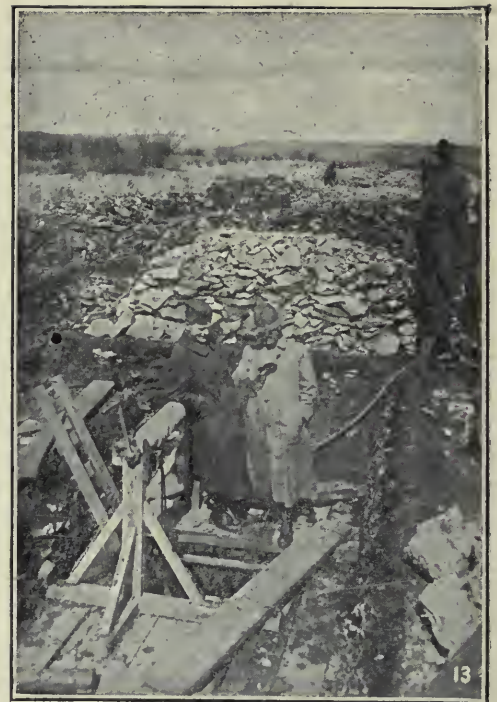
FIGS. 12 AND 13. THESE ARE THE ENTRANCES TO TWO MODEL DUGOUTS WHICH STUDENTS AT THE ARMY ENGINEER SCHOOL ARE EXCAVATING IN ROCK
