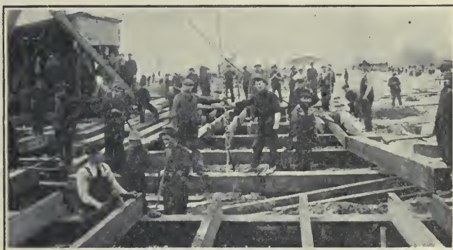
CONCRETING FLOORS OF CLASSIFICATION SHEDS
