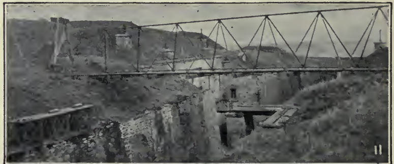
FIG. 9. FINISHING ERECTION OF LAST BENT—NOTE POSITION OF MEN, EACH HAVING SPECIFIC PLACE TO OCCUPY AT SPECIFIC TIME
