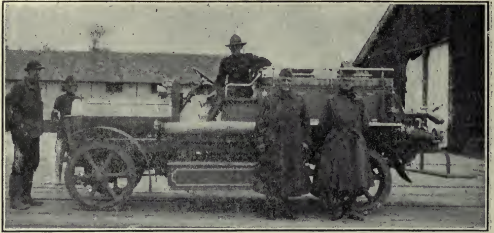
A. WOODEN DOCKS ARE PROTECTED BY MOTOR-DRIVEN FIRE-FIGHTING APPARATUS—IN FOREGROUND, MAJOR COMMANDING ENGINEER BATTALION AND CAPTAIN WHO HAD IMMEDIATE CHARGE OF DOCK CONSTRUCTION
