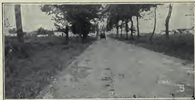
FIG. 5. FRENCH ROAD OF "GRANDE COMMUNICATION" TYPE—USE BY ARTILLERY IS PRODUCING RUTS AND HOLES WHICH WILL SOON NEED ATTENTION
