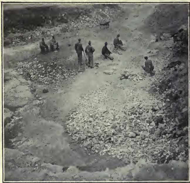
HAND QUARRYING PENDING ARRIVAL OF CRUSHER
