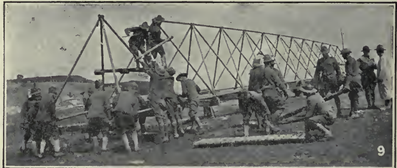
FIG. 5. BEFORE ERECTION AND LAUNCHING, PARTS OF THE LIGHT PORTABLE BRIDGE ARE LAID OUT ON THE GROUND PARALLEL TO LINE OF STREAM TO BE CROSSED
