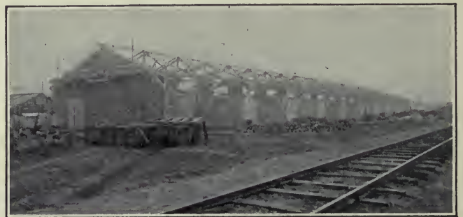
FIG. 2. WOOD-FRAME WAREHOUSE HAS HOLLOW TILE WALLS
