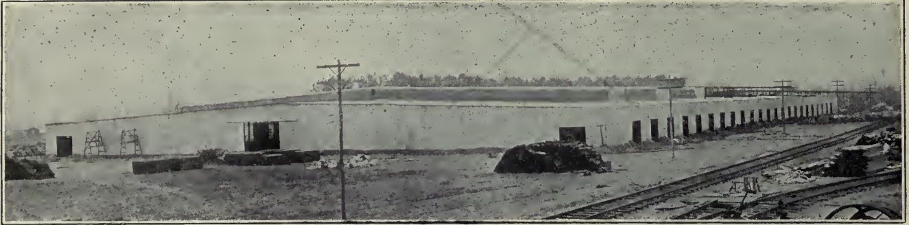
FIG. 6. ONE OF THE VERY LARGE STEEL FRAME WAREHOUSES SHEATHED WITH CORRUGATED IRON
