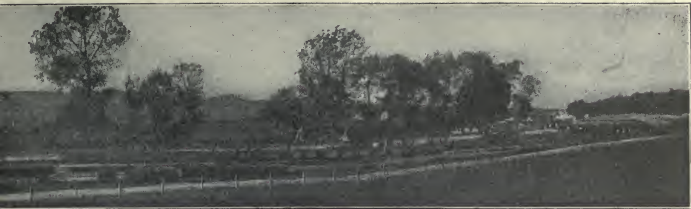
OF LIGHT-RAILWAY TRACK ALONG THE FRONT, IN BOTH THE FORWARD AND THE REAR AREAS
