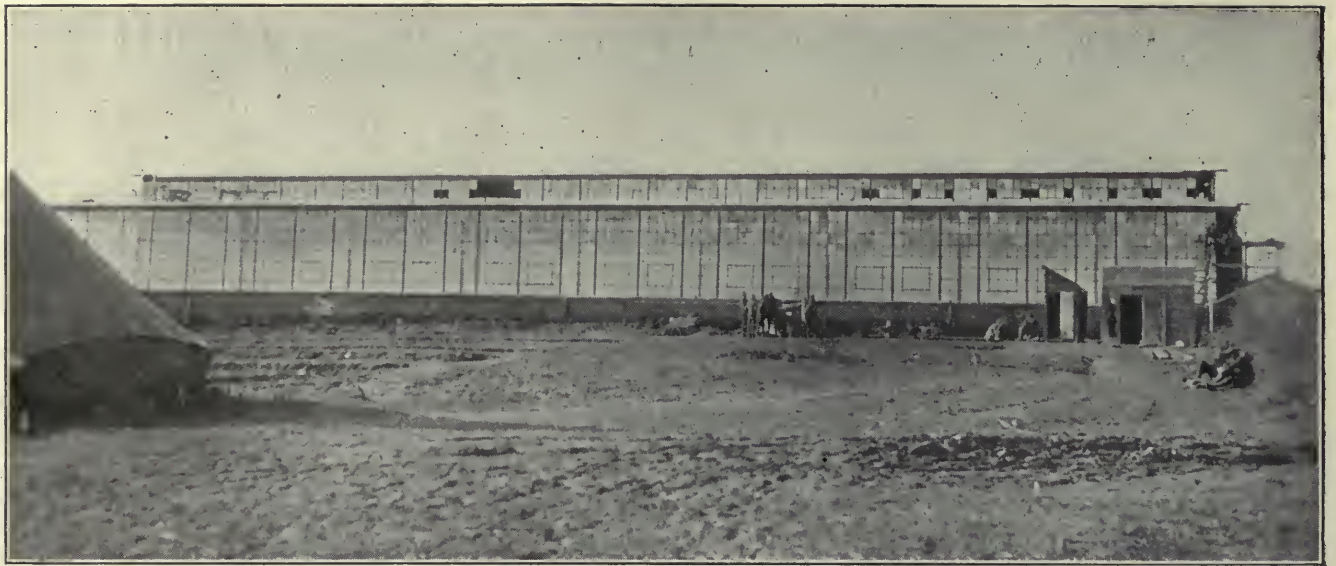
NEW AUTOMATIC ASSEMBLING PLANT IS STEEL FRAME STRUCTURE WITH GLASS SIDES AND MONITOR
