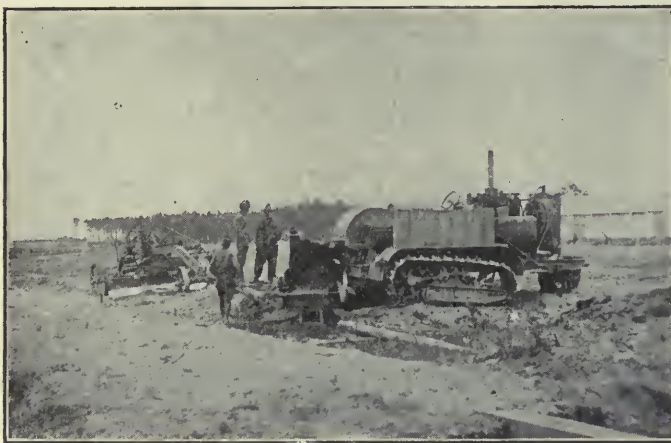
Photographs by Engineering News-Record FIG. 7. GRADING DONE BY AMERICAN ROAD GRADER HAULED BY CATERPILLAR, SHOWN ON LEFT, AND ROAD ROLLED BY AMERICAN MACHINE, IN VIEW AT RIGHT
