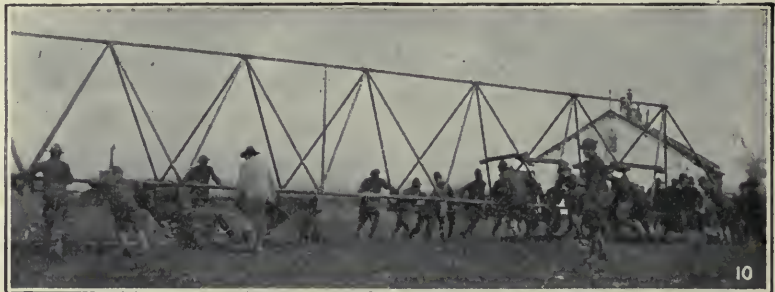
FIG. 7. THE FIRST BENT ERECTED AT ABOUT MIDDLE OF STRUCTURE, DIRECTLY OVER TWO-WHEEL TRUCK USED LATER FOR LAUNCHING
