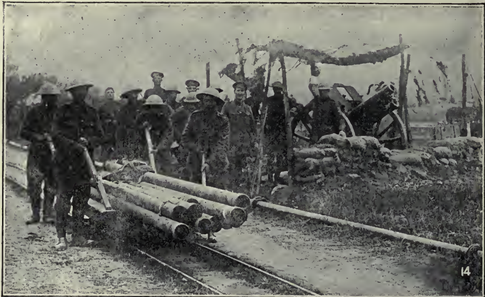
FIG. 14. BRINGING UP WATER PIPES TO SUPPLY THE FRONT LINE
