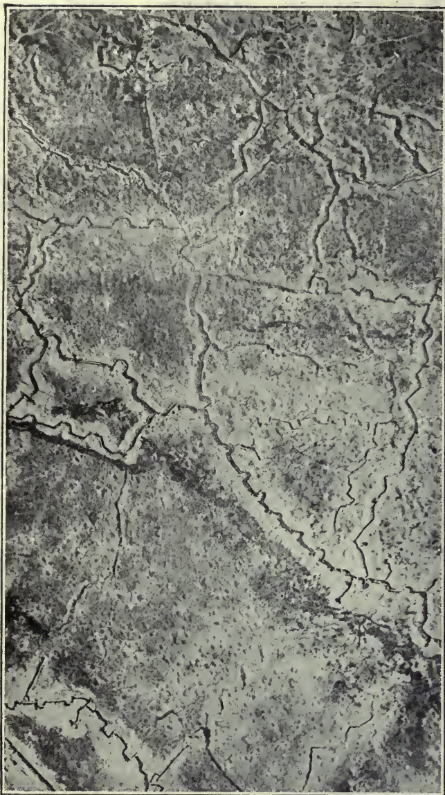
TRENCH SYSTEM SHOWS PLAINLY AT 1900 METERS
