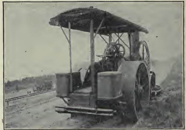
Photographs by Engineering News-Record FIG. 7. GRADING DONE BY AMERICAN ROAD GRADER HAULED BY CATERPILLAR, SHOWN ON LEFT, AND ROAD ROLLED BY AMERICAN MACHINE, IN VIEW AT RIGHT
