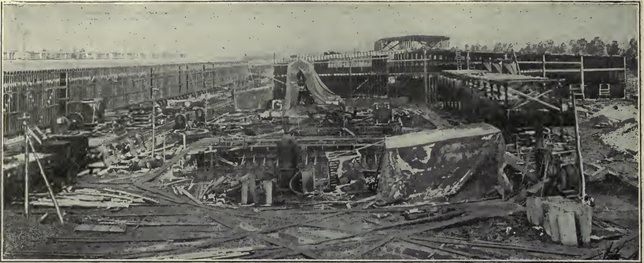
FIG. 10. REFRIGERATING PLANT UNDER CONSTRUCTION LAST WINTER
