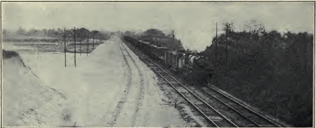
O. NEW RAILROAD, 6½ MILES LONG, LEADING FROM DEPARTURE YARD AT DOCKS TO BASE STORAGE DEPOT—NOTE GRADING FOR ADDITIONAL TRACKS
