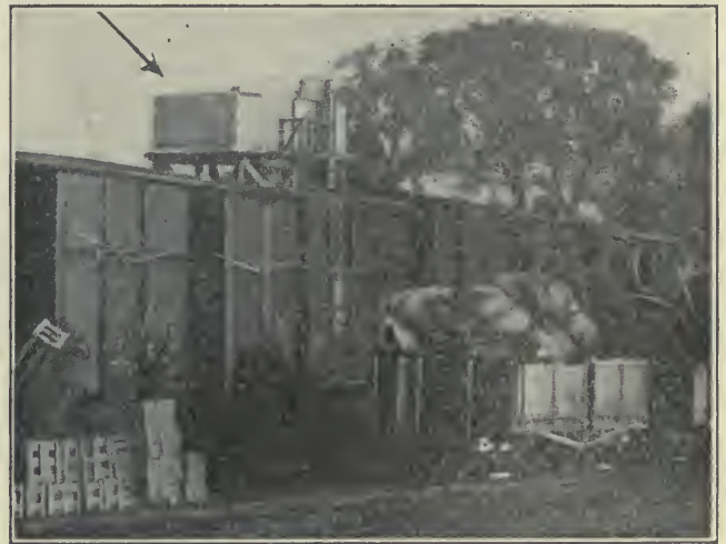
British Official Photo ELEVATED TANK (IN BACKGROUND, CENTER) FOR SUPPLYING WATER TO RAILWAY LOCOMOTIVES
