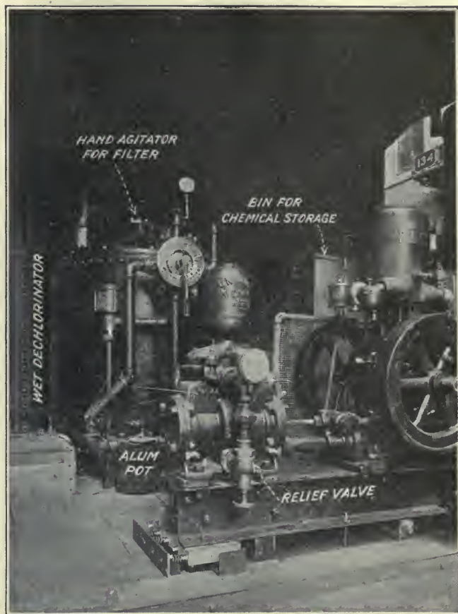
CORNER OF WATER ANALYSIS LABORATORY—PUMPING PLANT, PRESSURE FILTER AND DECHLORINATOR
