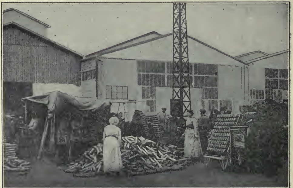
TRUCK REMOVING SHELL FORGINGS FROM AN INSPECTION POINT
