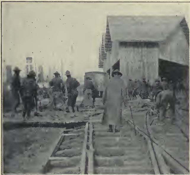
CONCRETE HAND-MIXED FOR NEW TRACK LAYOUT AT DOCKING BASIN
