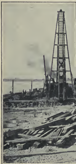
G. CAPPING PILES AND LAYING THE TIMBER DECKING AT THE AMERICAN DOCKS H. LOOKING ALONG DOCK SITE—PILEDRIVER ON LEFT, TIMBER CLASSIFICATION SHED IN CENTER J. THE ENGINEERS HAD TO BUILD THEIR OWN PILEDRIVERS AND DERRICKS
