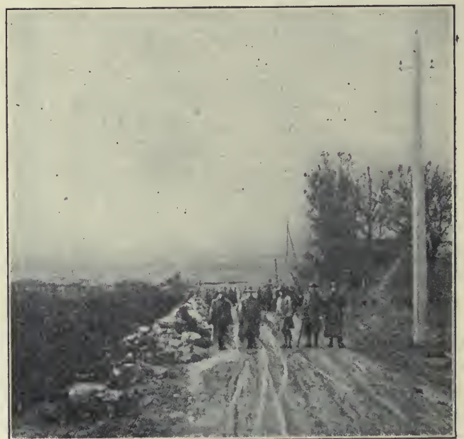
RIPRAP AT ROADSIDE WAITING FOR TRANSPORT TO EARTH DAM
