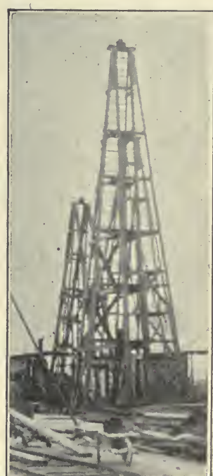
G. CAPPING PILES AND LAYING THE TIMBER DECKING AT THE AMERICAN DOCKS H. LOOKING ALONG DOCK SITE—PILEDRIVER ON LEFT, TIMBER CLASSIFICATION SHED IN CENTER J. THE ENGINEERS HAD TO BUILD THEIR OWN PILEDRIVERS AND DERRICKS
