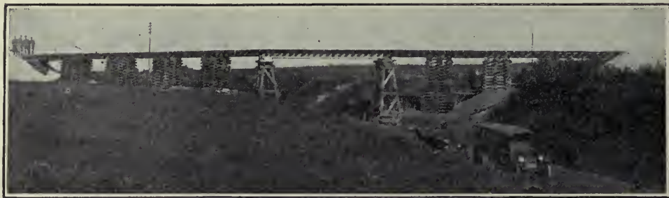
LIGHT RAILWAY CARS—OCCASIONALLY IT IS NECESSARY TO BUILD A TRESTLE
