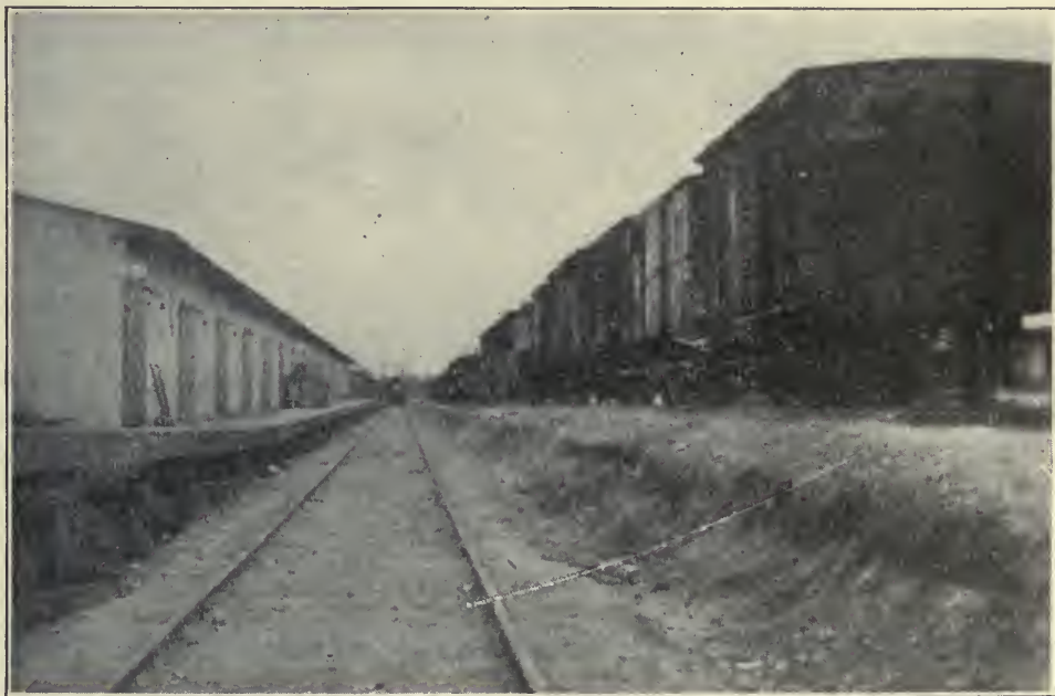
A. THE NINETEEN WAREHOUSES ARE EACH 500 x 250 FEET IN PLAN AND ARE ARRANGED IN SIX PARALLEL ROWS
