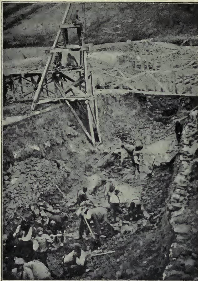
HAND DRILLING IN CUTOFF TRENCH FOR CONCRETE DAM
