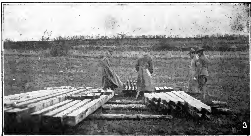
FIGS. 2 TO 4. AT ONE OF THE FIELDS OF THE ARMY ENGINEER SCHOOL MANY DIFFERENT TYPES OF PARTIALLY COMPLETED WOODEN BRIDGES ARE AVAILABLE FOR STUDY BY STUDENTS. IN FIG. 4 NOTE PARTICULARLY THE FORM OF ABUTMENT, WHICH CONSISTS OF CUBES OF STRUCTURAL STEEL BUILT UP LIKE BLOCKS
