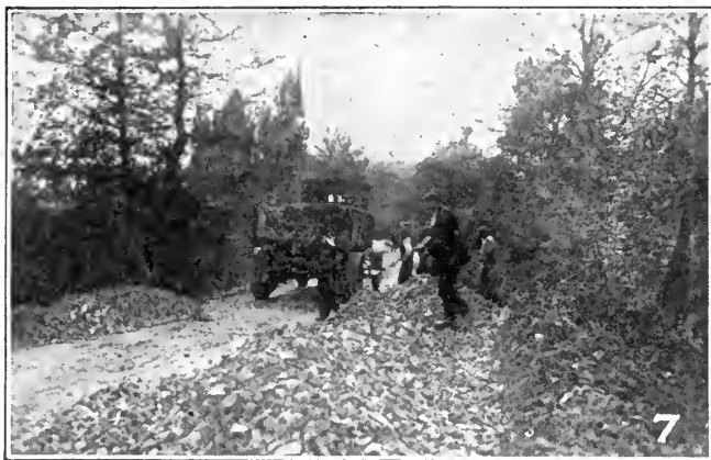
FIG. 6. 7 AND 8. WIDENING A NARROW ROAD LEADING INTO AN IMPORTANT AMERICAN ARMY CAMP — MOTOR TRUCKS DELIVER CRUSHED STONE TO THE JOB, AND THE STONE IS SPREAD ON EITHER SIDE OF THE ORIGINAL ROAD
