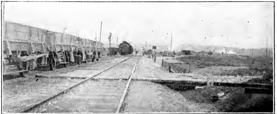
C. THE RAILWAY RECEIVING AND CLASSIFICATION YARDS ARE THE WORK OF AMERICAN ENGINEERS
