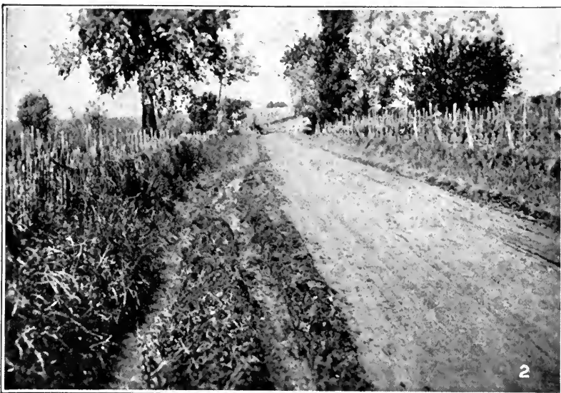
FIGS. 1 AND 2. TWO VIEWS ALONG FARM ROAD THREE METERS WIDE NOW BEING USED BY OUR FIELD ARTILLERY TROOPS FOR PRACTICE MARCHES — NOTE MARKS LEFT BY CATERPILLAR TREADS OF BIG GUN CARRIAGES AND NOTE ALSO HOW TRAFFIC HAS BEEN FORCED OUT ON SHOULDERS AND INTO DITCHES
