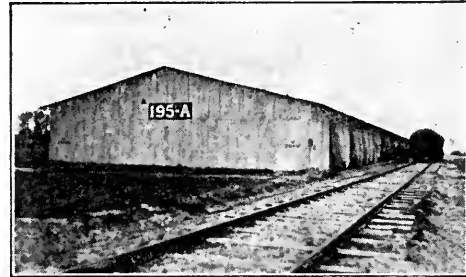
FIG. 4. ENDS OF WOOD-FRAME WAREHOUSES ARE SHEATHED WITH CORRUGATED IRON BUT SIDES HAVE ONLY CANVAS COVERS
