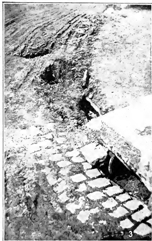
FIGS. 1 AND 2. TWO VIEWS ALONG FARM ROAD THREE METERS WIDE NOW BEING USED BY OUR FIELD ARTILLERY TROOPS FOR PRACTICE MARCHES — NOTE MARKS LEFT BY CATERPILLAR TREADS OF BIG GUN CARRIAGES AND NOTE ALSO HOW TRAFFIC HAS BEEN FORCED OUT ON SHOULDERS AND INTO DITCHES
