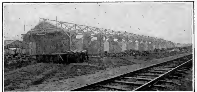
FIG. 2. WOOD-FRAME WAREHOUSE HAS HOLLOW TILE WALLS
