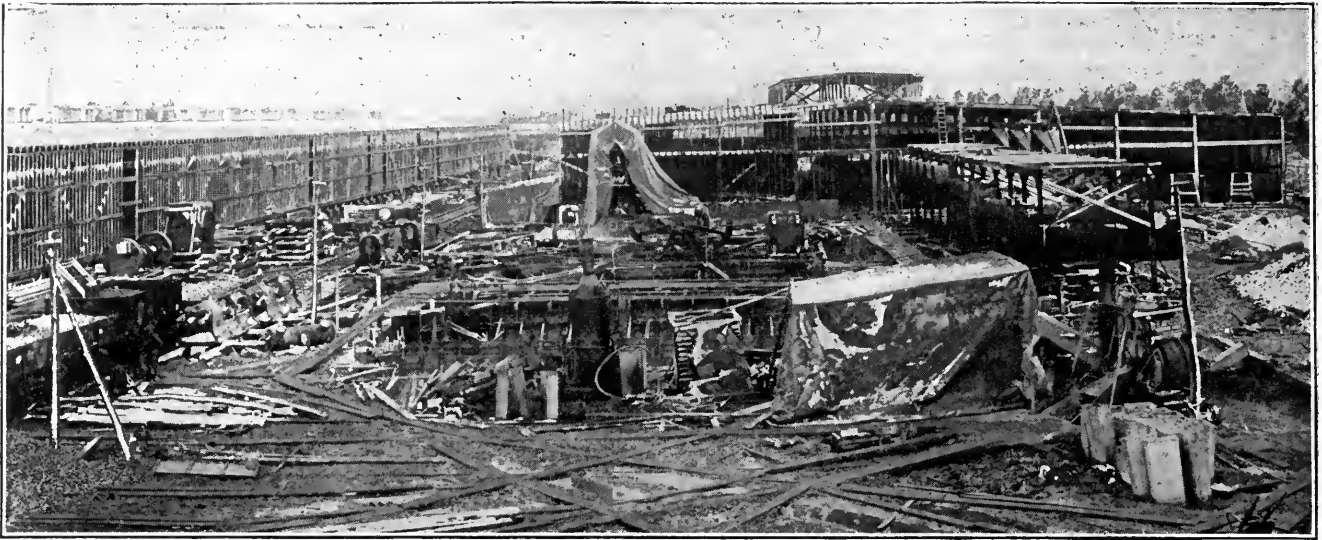
FIG. 10. REFRIGERATING PLANT UNDER CONSTRUCTION LAST WINTER
