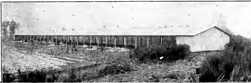
FIG. 4. ENDS OF WOOD-FRAME WAREHOUSES ARE SHEATHED WITH CORRUGATED IRON BUT SIDES HAVE ONLY CANVAS COVERS
