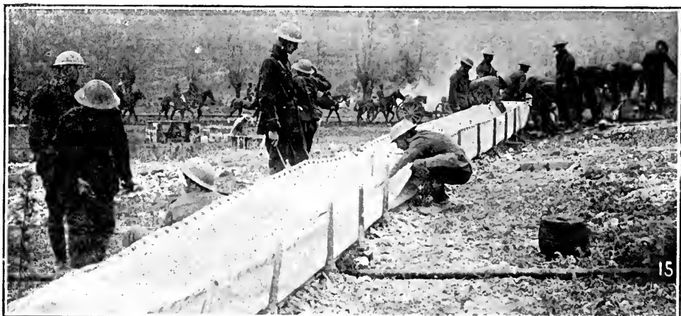
FIG. 15. PUTTING UP A WATER TROUGH FOR THE CAVALRY
