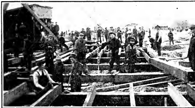
CONCRETING FLOORS OF CLASSIFICATION SHEDS
