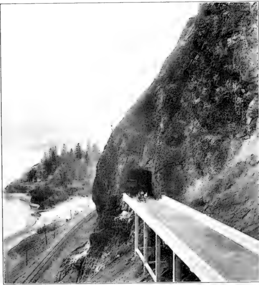
THE APPROACH TO A TUNNEL
