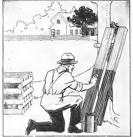
Showing application of Grade-One Creosote Oil by hand.
