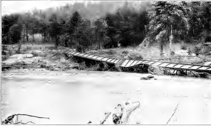
IRON GIRDERS CARRIED AWAY BY FLOOD
