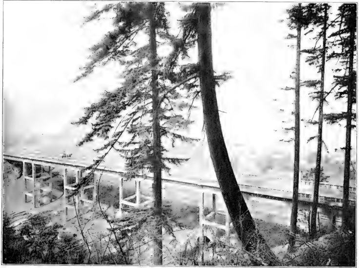
MCCORD CREEK BRIDGE
