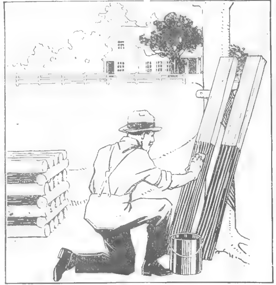
Showing brush application by hand of Carbosota—Barrett's Grade-One Creosote Oil.
