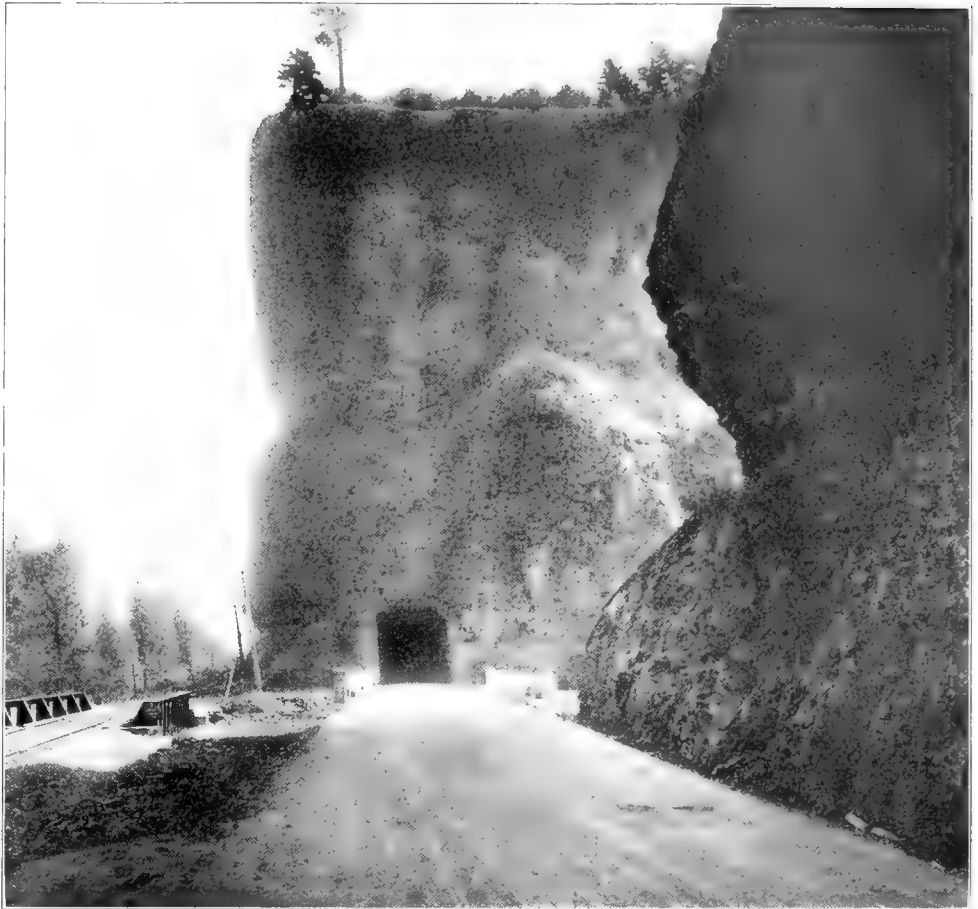
ANOTHER TUNNEL AND BRIDGE
