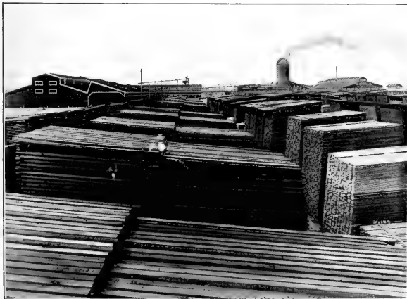
A LARGE AIR-DRYING YARD OF DOUGLAS FIR
