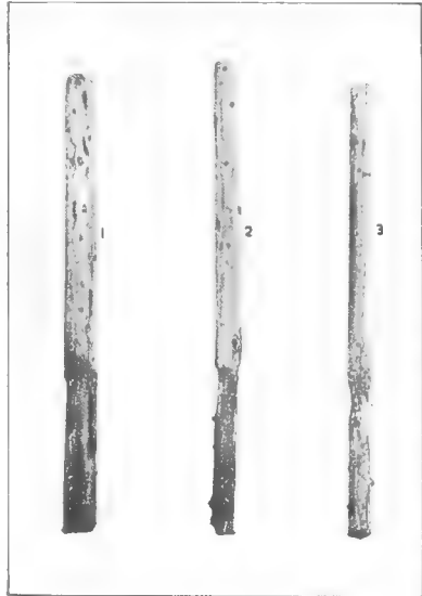
Untreated. These Cedar posts were set in 1905 and taken up for examination in October, 1914. In each case the sap-wood was entirely gone; in post No. 1 about one-third of the entire bottom rotted away; in post No. 2 one-half of the bottom decayed.
