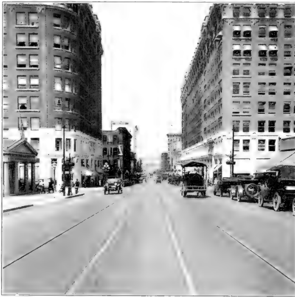
A CREOSOTED DOUGLAS FIR WOOD BLOCK PAVEMENT
