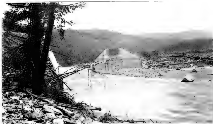
C. C. AND O. R. R. BRIDGE DEMOLISHED
