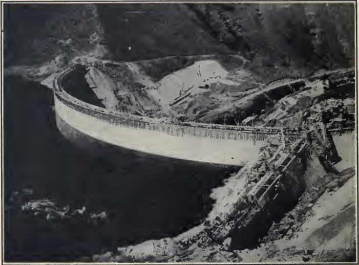
ARROW ROCK DAM, IDAHO, UNDER CONSTRUCTION.
