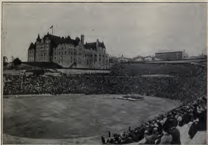
HIGH SCHOOL AND STADIUM, TACOMA, WASHINGTON.
