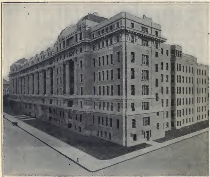
COOK COUNTY HOSPITAL IN CHICAGO.
