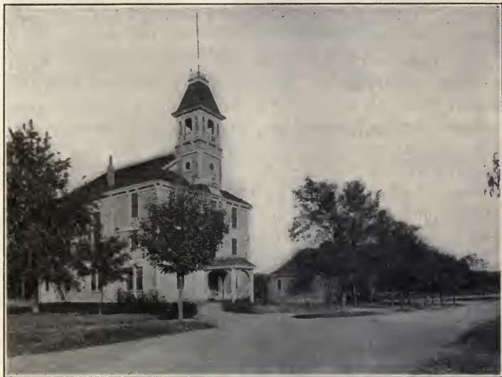
TOWN HALL, DOVER, MASSACHUSETTS.
