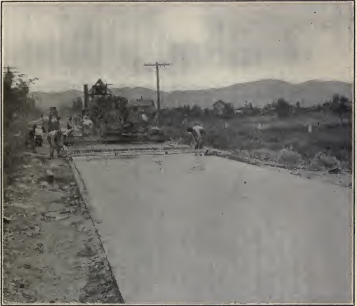
ROAD BUILDING ON THE PACIFIC HIGHWAY, OREGON.
