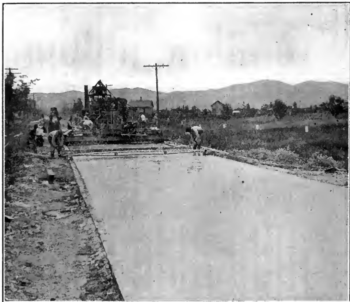
ROAD BUILDING ON THE PACIFIC HIGHWAY, OREGON.
