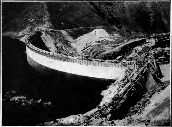
ARROW ROCK DAM, IDAHO, UNDER CONSTRUCTION.
