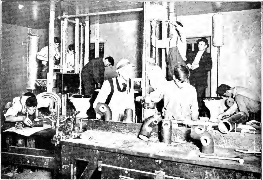
INDIANS RECEIVING INSTRUCTION IN PLUMBING. HASKELL INSTITUTE, KANSAS
