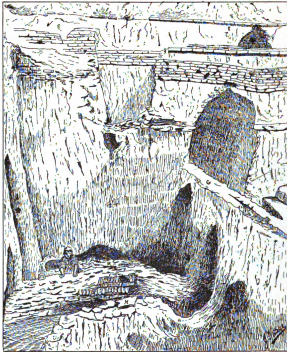
FIG. 46.—EXCAVATIONS ABOUT AND ABOVE THE ARCH.
