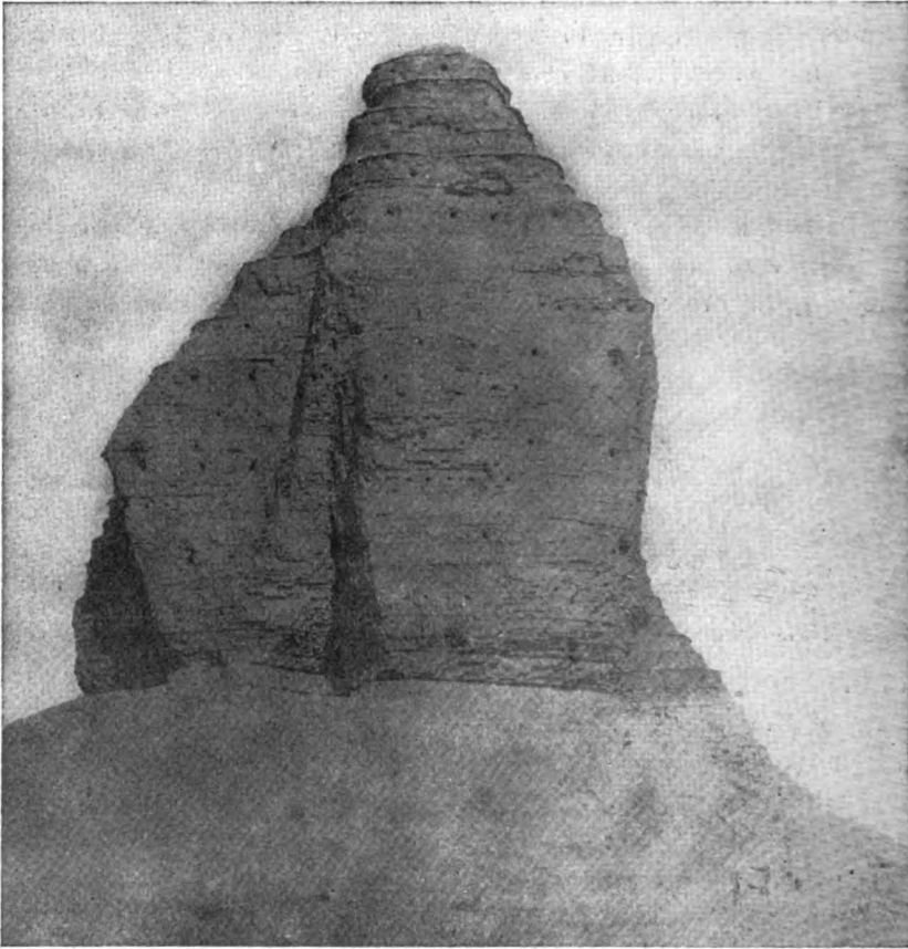
FIG. 67.—RUINS OF TOWER AT AKER KUF.
