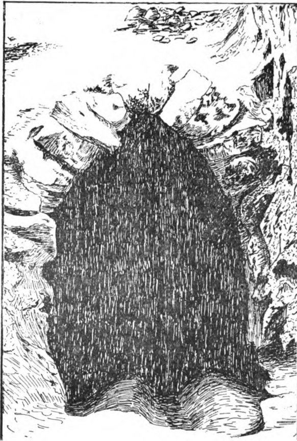
FIG. 41.—VIEW OF ARCH FROM THE INSIDE.
