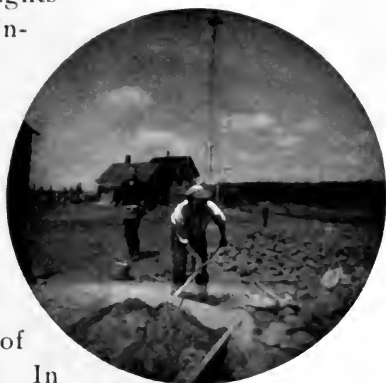
MIXING MORTAR
