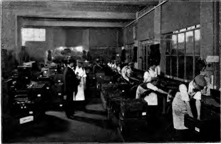
FIG. 5.—THE INSPECTION ROOM
